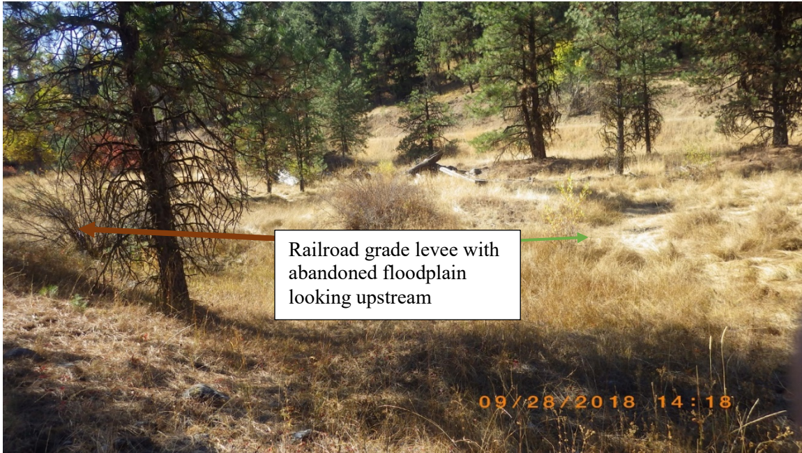
Figure 11 General characteristics of abandoned/separated floodplain due to railroad grade levee, Camp Creek reach 5
