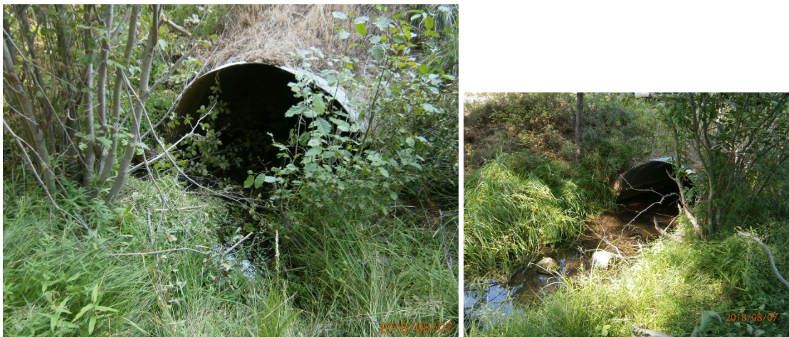
Figure 19. National Forest System Road 2622 culvert on Idaho Creek
