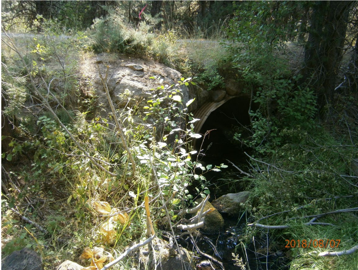
Figure 16. National Forest System Road 1940281 Culvert on Summit Creek
