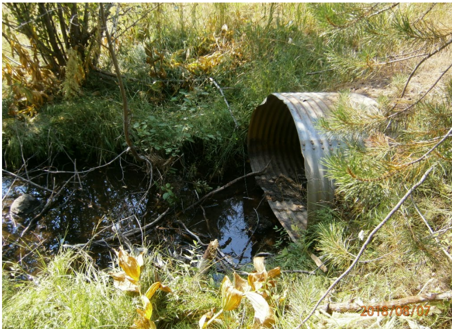
Figure 14. National Forest System Road 1940 culvert outlet on Summit Creek
