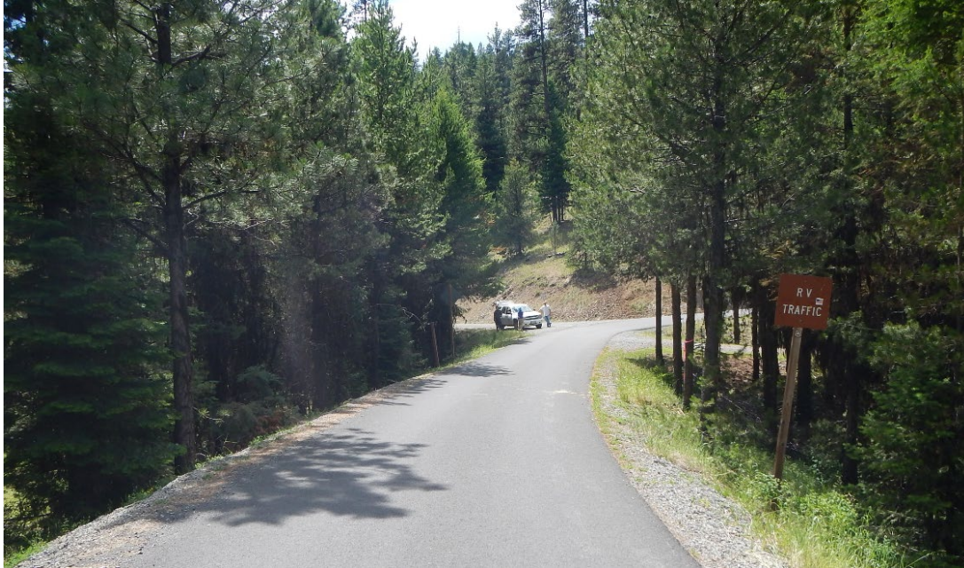
Figure 4. National Forest System Road 3620 that culvert will be replaced on
