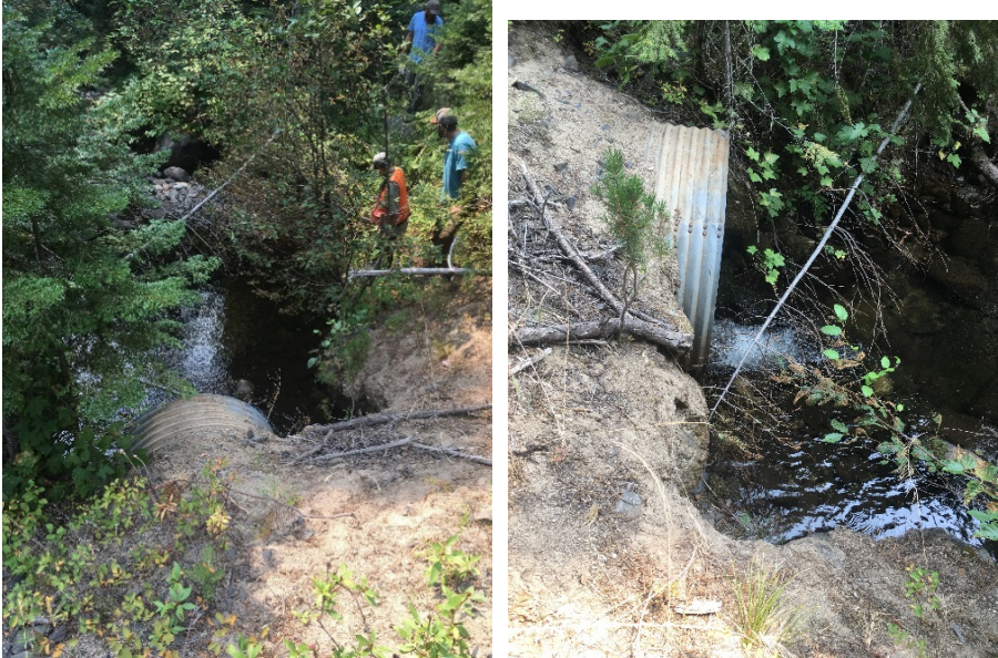
Figure 24. National Forest System Road 4560 culvert on Deadwood Creek (outlet)
