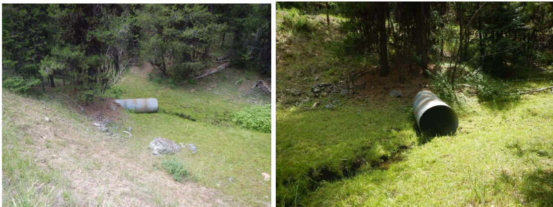
Figure 6. Existing Tinker Creek culvert inlet, alignment and culvert size
