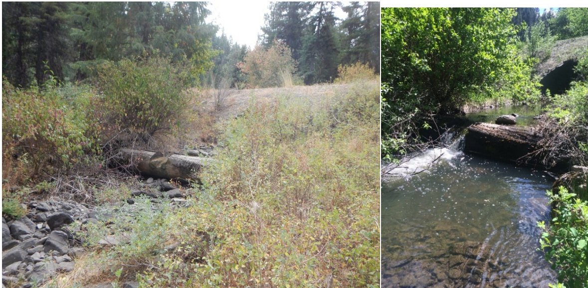
Figure 8. National Forest System Road 36 log weir in downstream of culvert on Cottonwood Creek (right photo: taken 5/17/2016)
