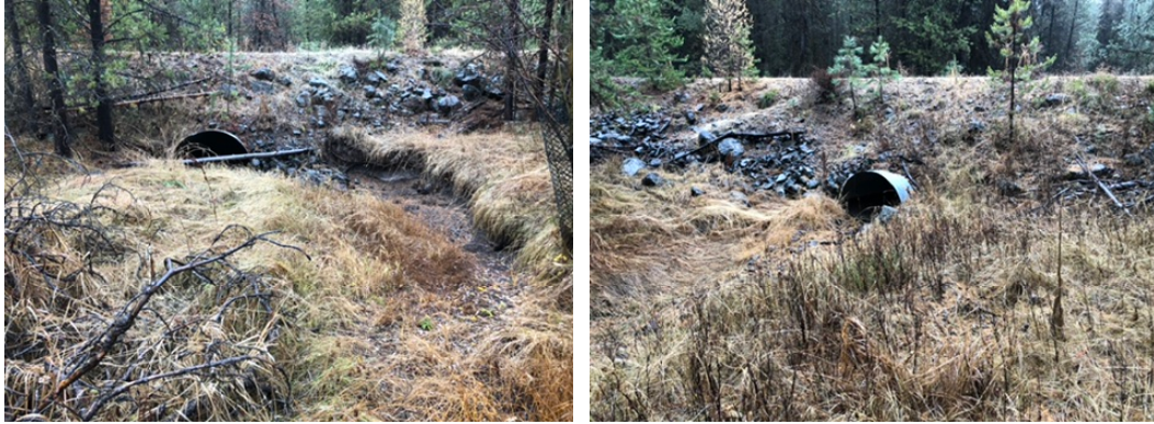
Figure 17. National Forest System Road 2622 culvert on Summit Creek
