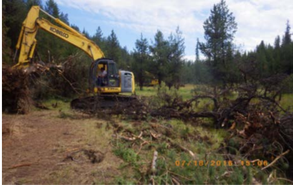
Figure 5. Excavator placing small wood (lodgepole pine) within overflow channel of Camp Creek in 2016
