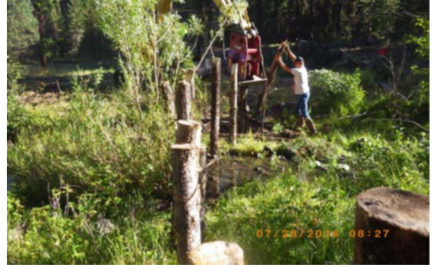
Figure 7. Excavator with compactor head driving posts for beaver dam analogue structure in Camp Creek in 2016
