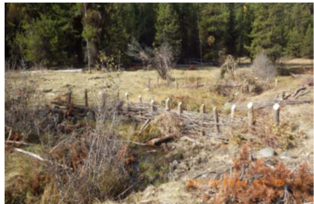
Figure 8. Beaver dam analogue with willow weaves prior to sealing in Camp Creek in 2016
