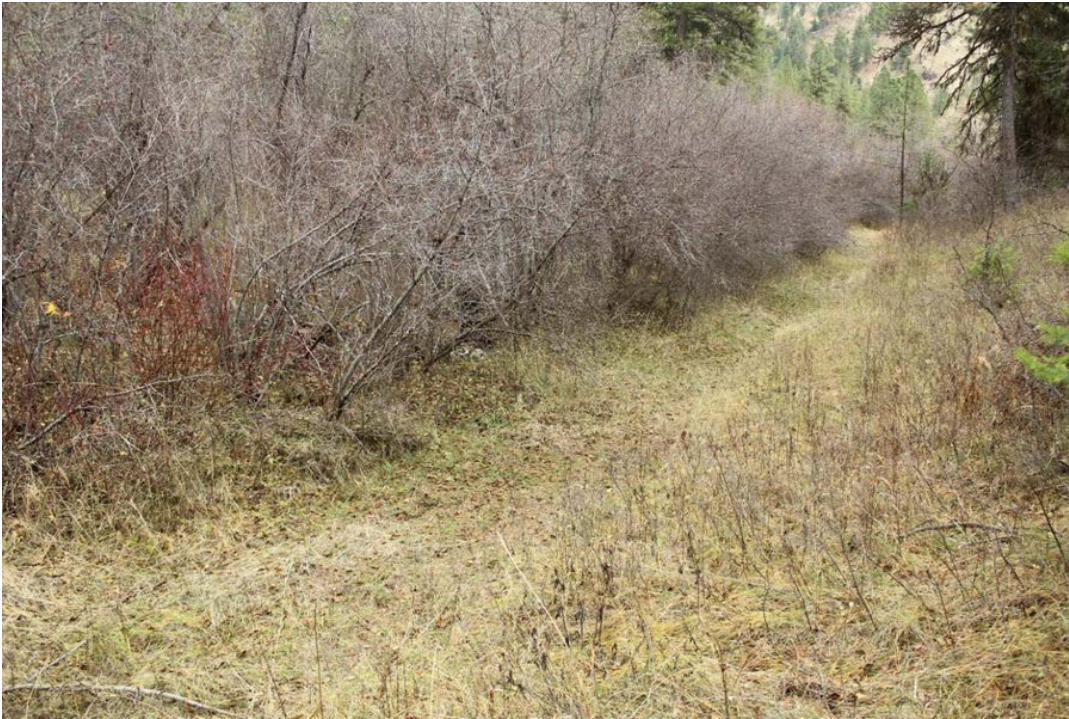
Figure 4. This berm, associated with the construction of National Forest System Road 36900018 (visible running from left bottom to right mid-ground), constricts Bear Creek from being able to access its entire floodplain. Under this proposal, the berm would be removed or breached and the roadbed scarified and seeded with native grasses.
