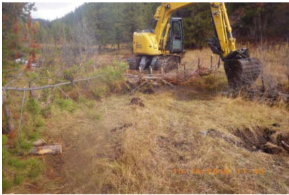
Figure 6. Excavator with wide bucket for scraping sedge mats, substrate, and soil related to beaver dam analogue sealing over willow weaves in Camp Creek in 2016
