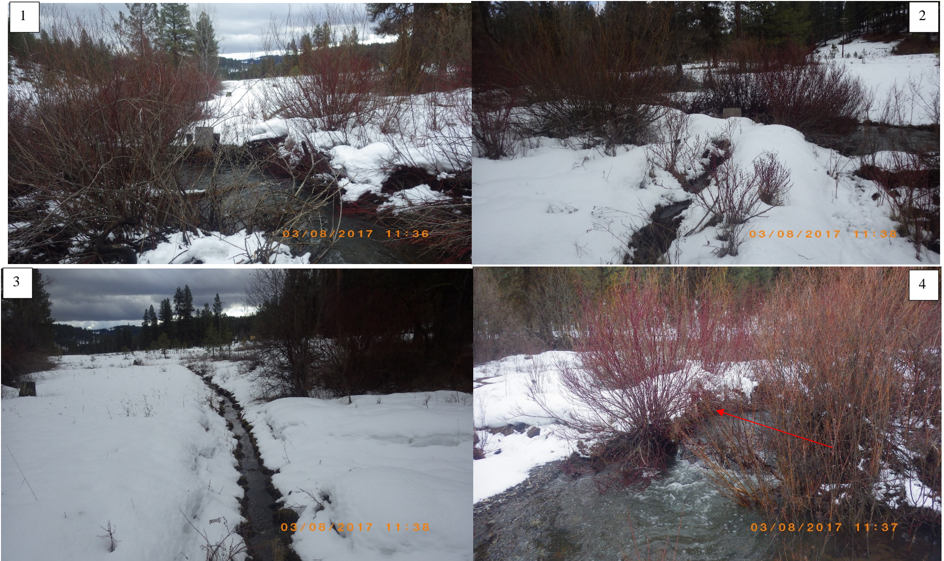
Figure 6. Beech Creek Diversion- 1) Looking downstream at point of diversion, 2) looking upstream at point of diversion 3) point of diversion looking down ditch, 4) point of diversion looking upstream Beech creek.
