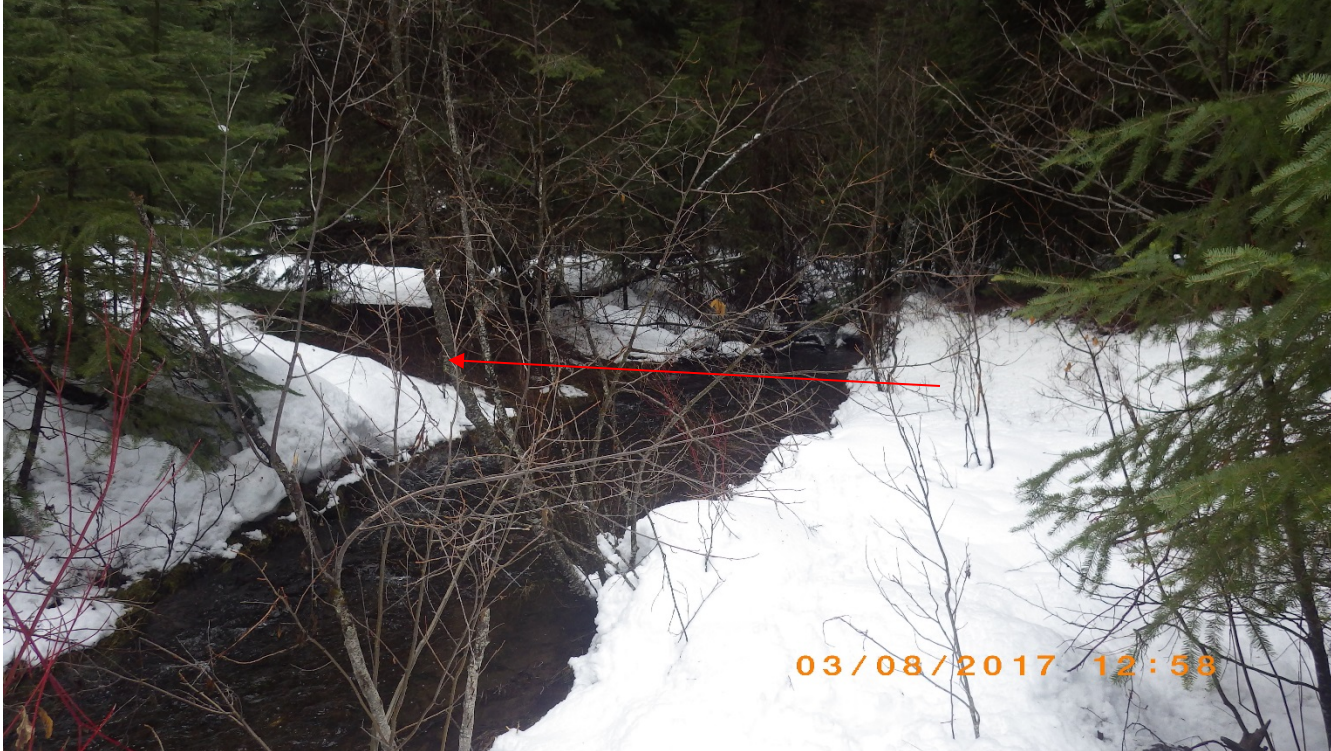
Figure 8. Bear Creek Diversion- 1) looking downstream at point of diversion, 2) looking down ditch from point of diversion, 3) looking downstream at point of diversion
