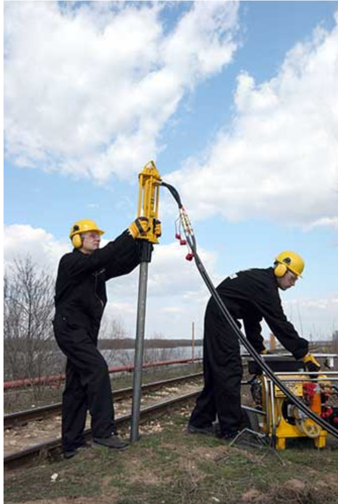
Figure 6 Hand held hydraulic post pounder with power pack used for placing posts (BDAs, Picket Baffle)
