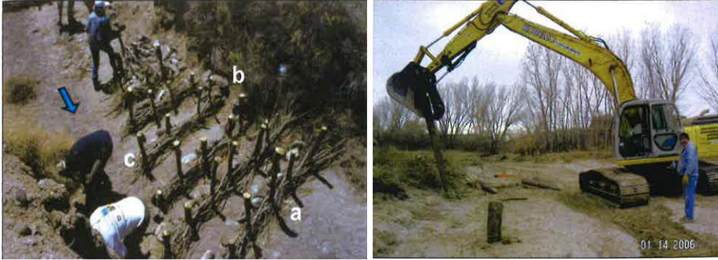
Figure 3 Illustration of a picket baffle with willow weave and an excavator placing posts
