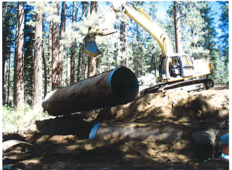
An excavator or backhoe will be used to remove problematic culverts
