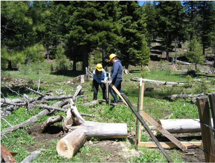
Representative riparian fencing will incorporate standing trees for fence posts and may include tree thinning to accelerate maintenance
