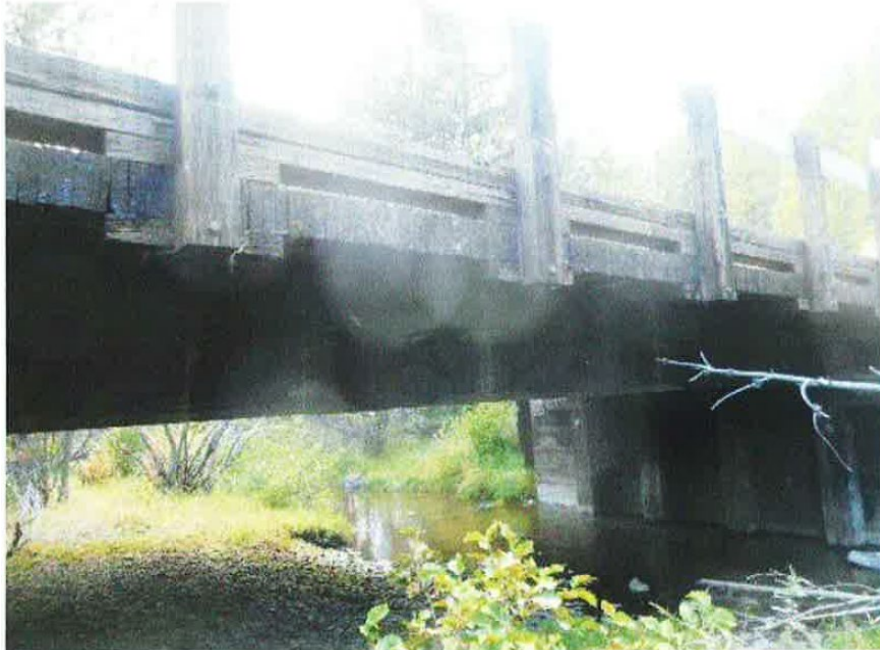
Figure 5. Summit Creek Bridge, looking downstream.
