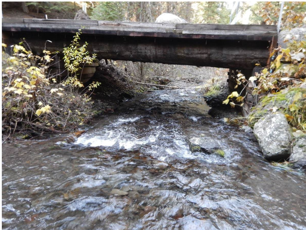
Figure 6. Bogue Gulch Bridge, looking downstream.
