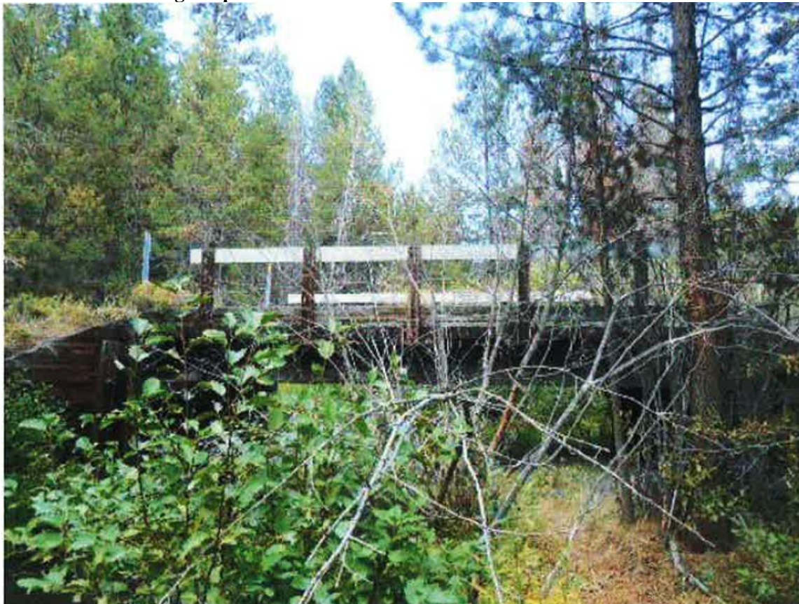
Figure 4. Summit Creek Bridge, looking upstream.
