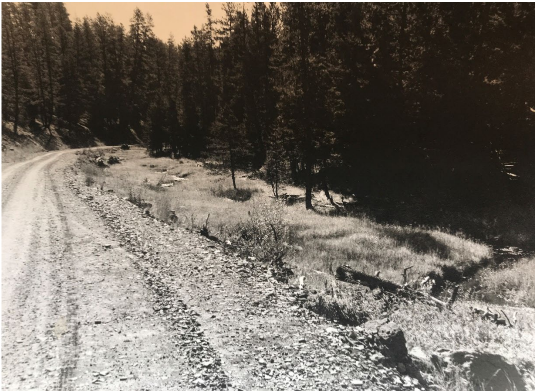
Figure 10. Photo of the same reach in 1965. The road grade has been expanded and Crane Creek has incised several feet, developing a single-thread channel with very little roughness within the valley bottom.
