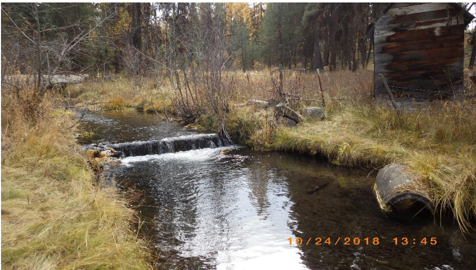
Figure 4: Typical log weir installed on Clear Creek within project area. The jump height on this weir is reduced but two other weirs in close proximity to this location have jump heights greater than 12”. Note the legacy water development infrastructure on the floodplain immediately adjacent to the stream.
