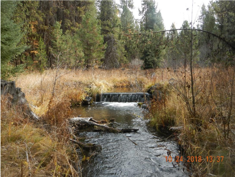
Figure 3: Typical log weir installed on Clear Creek within the project area, note the ~15-18” jump height, over-widened and straightened channel form downstream of the structure and riprap berms on both stream banks holding the log in place.
