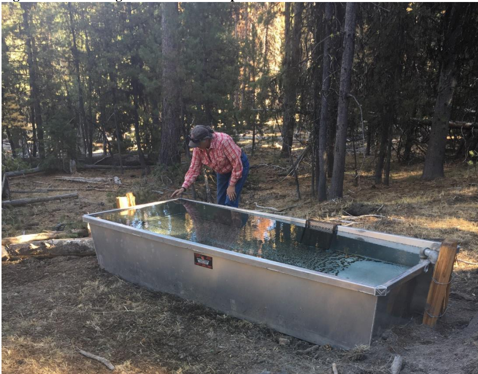
Figure 19. New trough installation example
