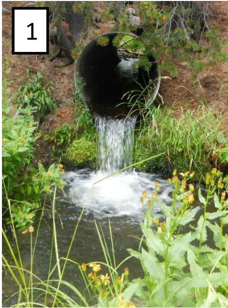
Figure 3 existing conditions of problem culverts; 1) Summit Creek @ 6200598 road, 2) North Summit Creek & 6200000 road, and 3) West Summit Creek @ 6200135 road.
