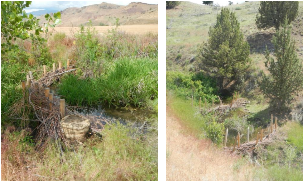
Figure 3. Examples of Beaver Dam Analogues in Pine Creek, a tributary to the John Day River near Fossil, OR, using fence posts which were installed with a manually operated hydraulic post-pounder.
