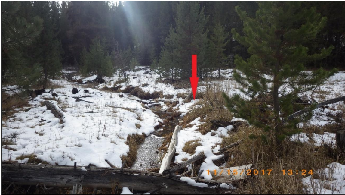
Figure 3. Facing upstream at current point of diversion, existing ditch is identified with red arrow.
