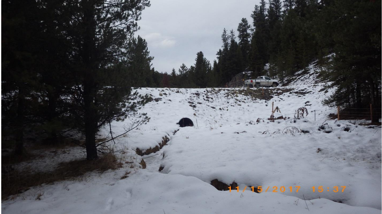
Figure 4: Existing culvert on FSR 2645-104 facing downstream.
