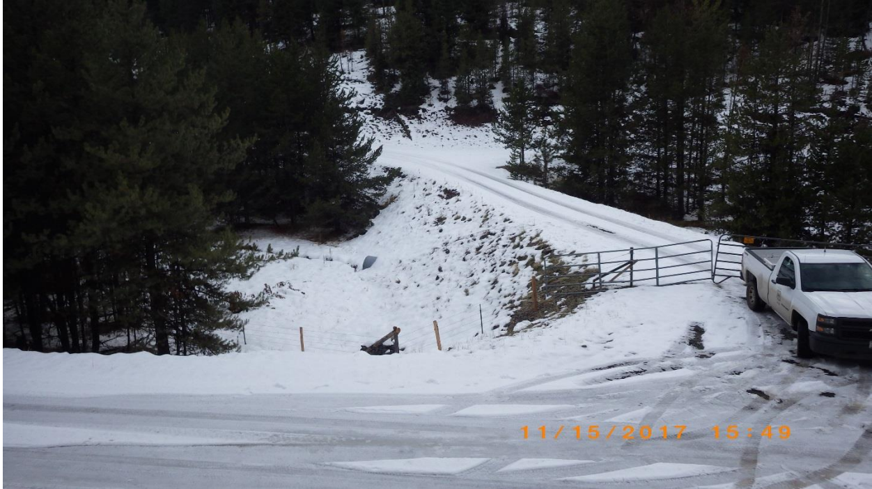
Figure 2: General site overview of proposed culvert replacement location on FSR 2645-104.
