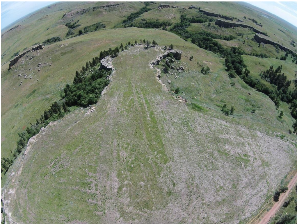
8. Reclaimed Western Portion of Bluff I (i.e. Bluff I2) (Photo taken in July 2015)
