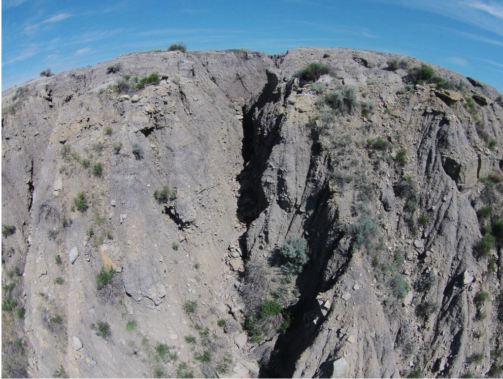
1. Bluff B Drainage (Photo taken in July 2015)
