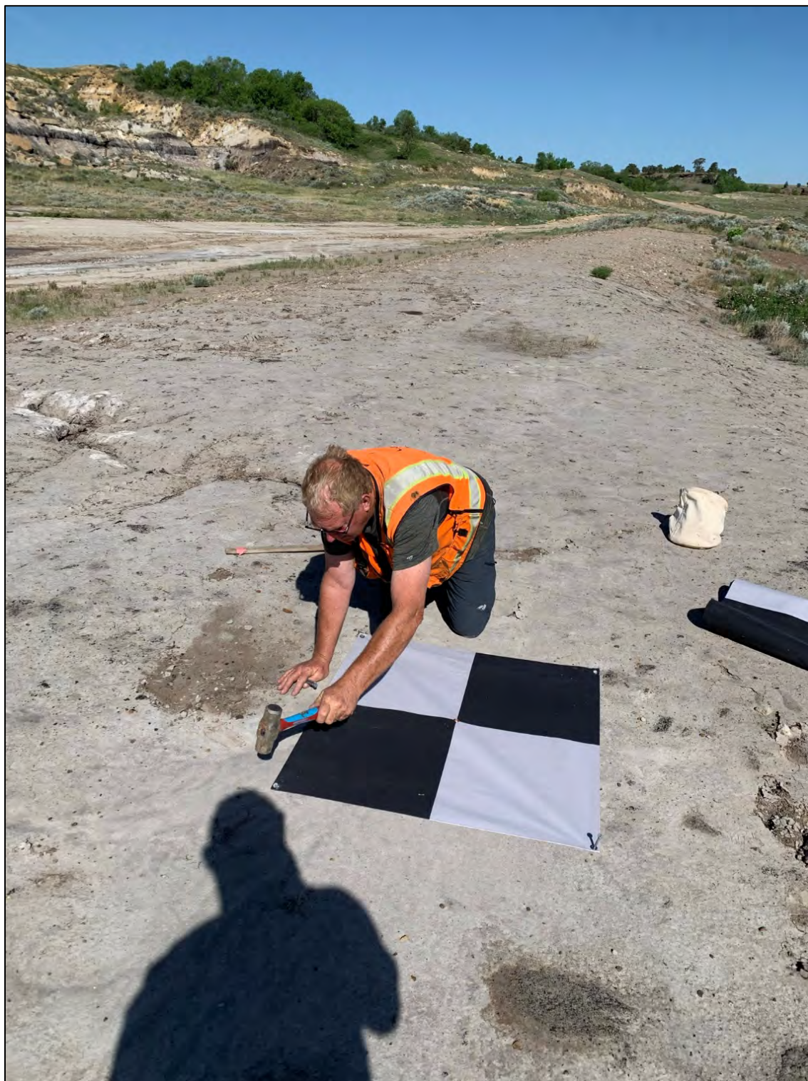
Photo 1 Setting Up Control Target for UAV Photogrammetry Survey
