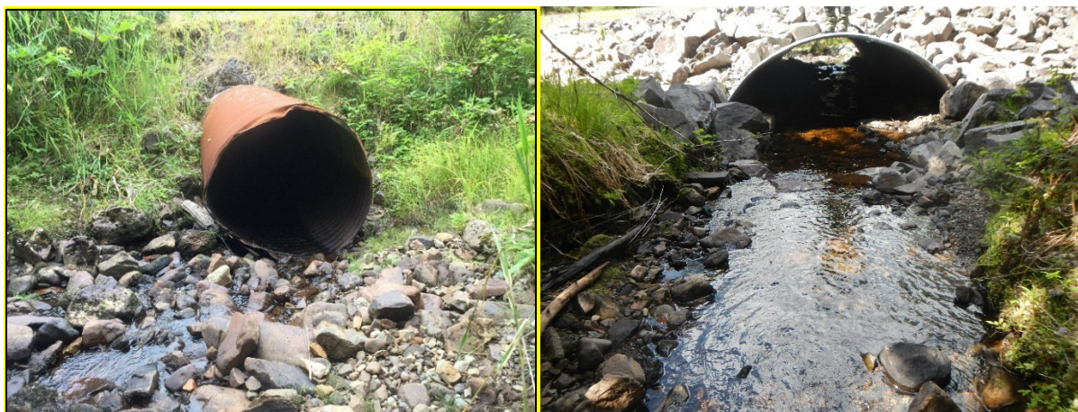
Figure 2: Before and after picture of recently replaced red pipe that was monitored in 2021. Looking downstream at culvert inlet.
