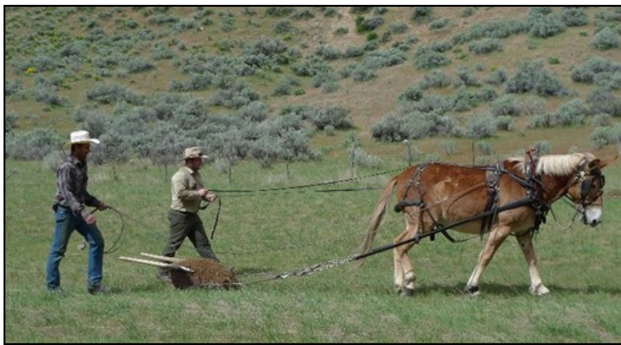
Getting fill material for Bernard airstrip on the Salmon-Challis National Forest.
