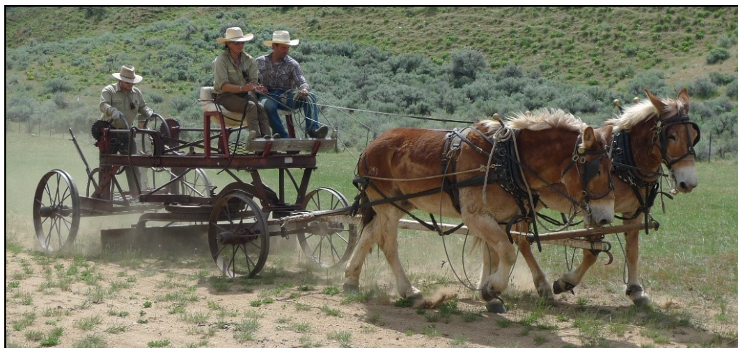
2018 grading work in progress on Bernard Airstrip.
