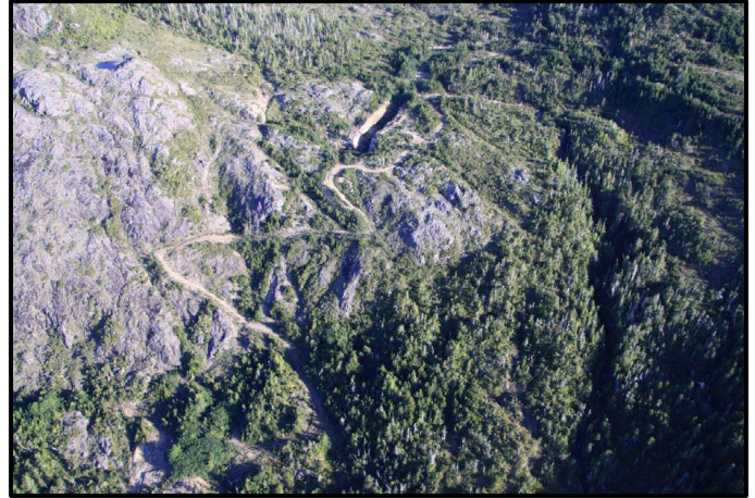
Ross Adams Mine aerial view.
