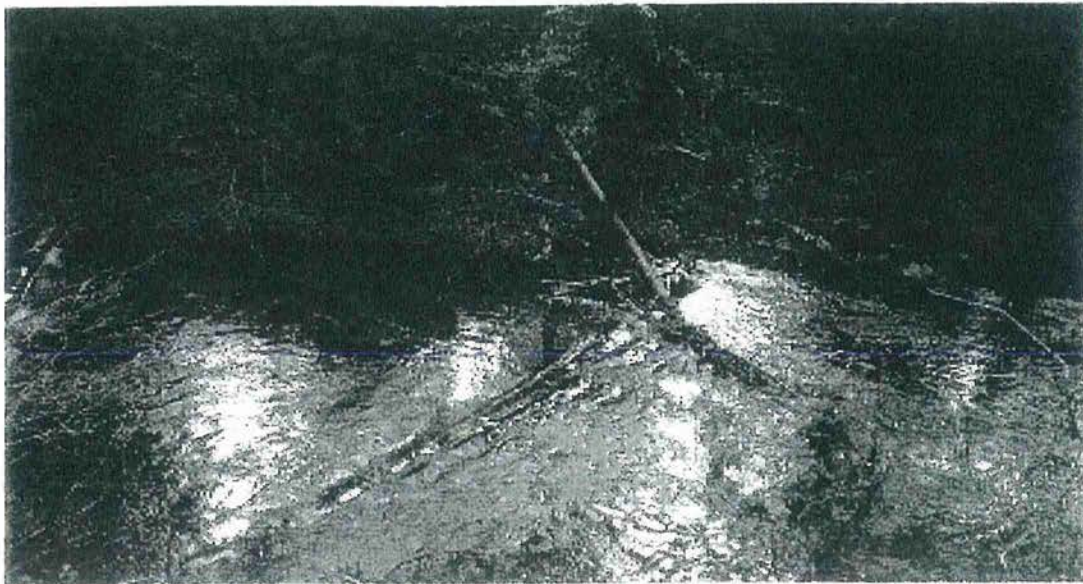
Blue River aquatic ecosystem restoration project photopoint monitoring. Photopoint 2 taken autumn 1993. Notice logs attached to bare bedrock. The wood was placed on bedrock in summer 1993.
