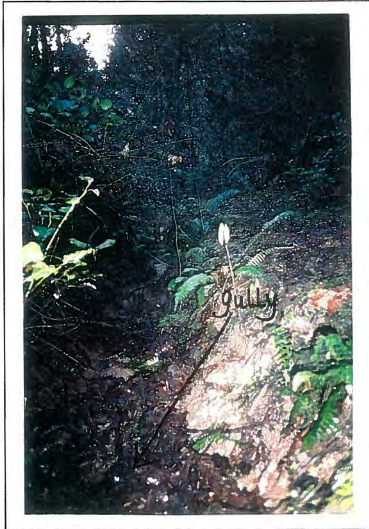
PHOTO CMB1. Photo of a gully in the tread of an abandoned road in the headwaters of Cedar Creek/Hills Creek drainage.
