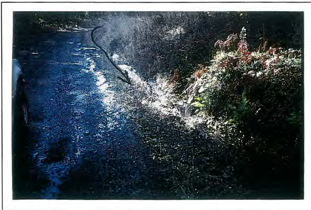
PHOTO CMB2. Flow diverted into ditchline with a long infeed length along Hills Creek mainline.
