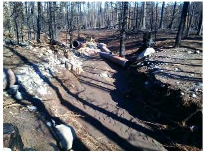
Post-fire- Road 1526-200 After storm event which overtopped culverts and washed out road bed
