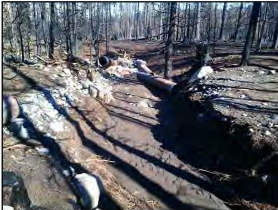
Washout of Rd 1526-200 after a storm event in the Pole Creek Fire Area
