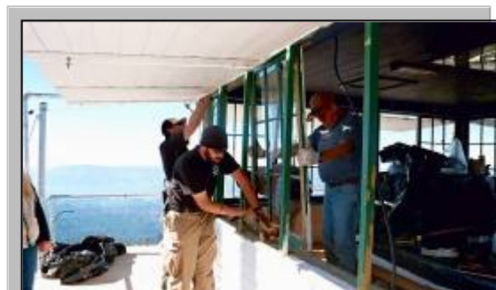
Forest workers remove the Scott Mountain Lookout's original 1930s windows, preparing them for rehabilitation.
