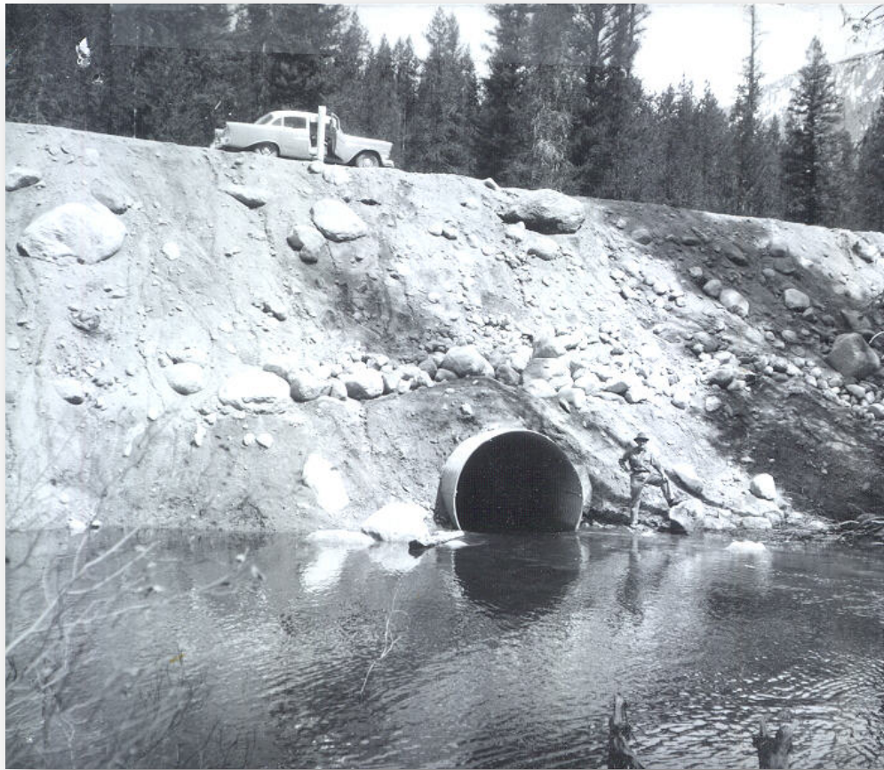
Newly Installed Goat Creek Culvert, South Fork Salmon River, 1955.
