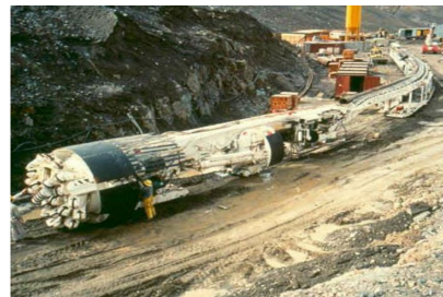
Tunnel boring machine
