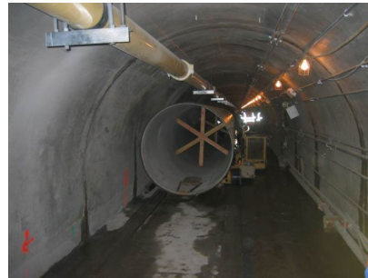
Example new tunnel construction
