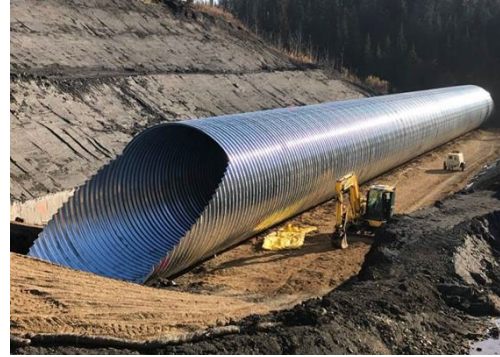
Example buried conduit installation
