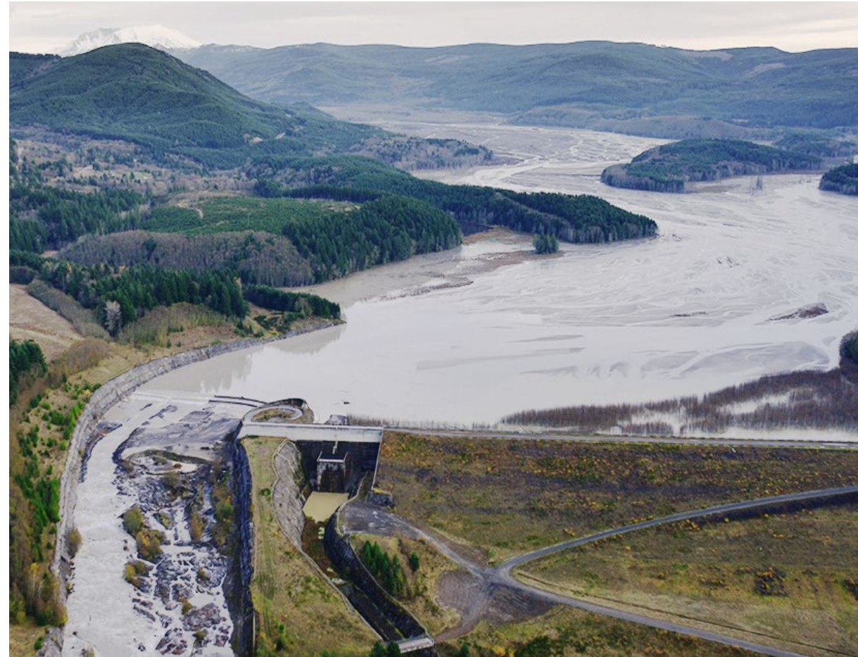
USACE Sediment Retention Structure on the North Fork Toutle River (Photo Credit: USACE)
