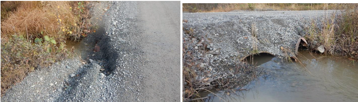
Figure 3: Inlet (Left) and outlet (Right) of SHER 3 in 2017.
