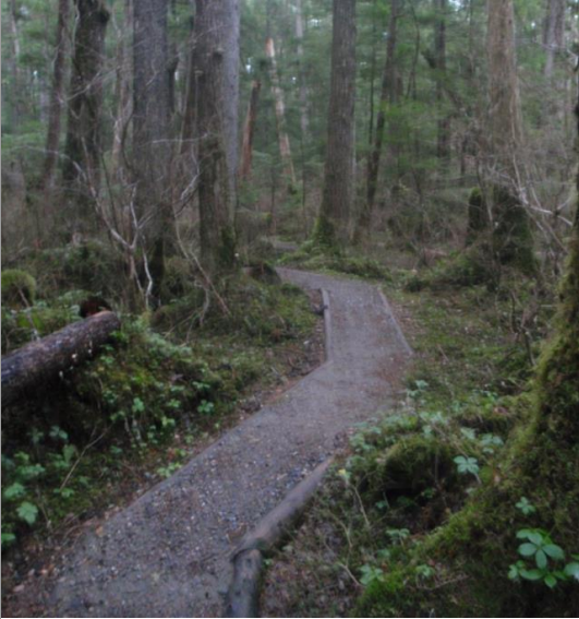
Figure 2: This picture shows a trail construction similar to that being proposed for the trail to The Claw. Four inch logs will border compacted D1.
