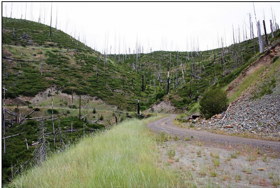
Figure 43 – Camera point 10, view 1 (upper image, June 1997; lower image, July 2008). This view looks north into headwaters of Lick Creek from 5507 road, about ¼ miles below its upper junction with 5510 road. In upper image, many trees have scorched foliage, suggesting that perhaps a few of the ponderosa pines might survive their fire effects (depending on time-of-burn, prefire moisture conditions, and other factors, ponderosa pines are known to occasionally survive very high amounts of crown scorch because their terminal branch buds are well protected). As has been consistently noted in this report, however, lower image shows that none of these trees survived.
