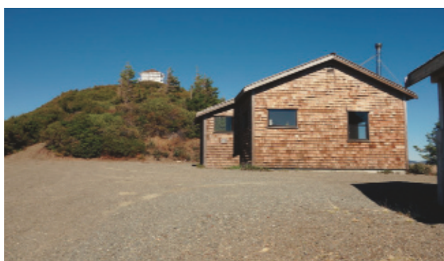
Lookout, cabin, parking area, and eave of toilet building
