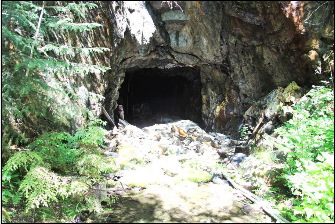
Photograph of 300-Foot Level Portal
