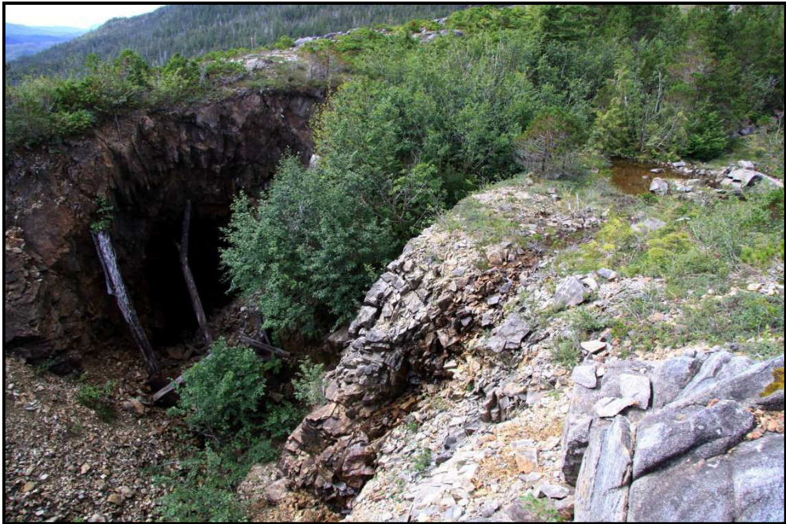
Photograph Looking Southwest Down into the Open Pit and 900-Foot Level portal showing the point at which surface runoff from the north and west (seen on the right side) enters the pit. (Note: Flow at the time the photo was taken was on the order of several gallons per minute.)
