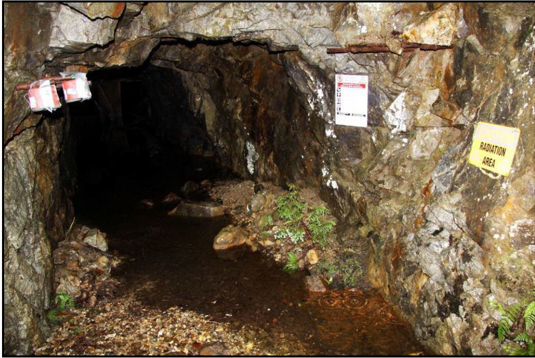
Photograph of 700-Foot Level Portal
