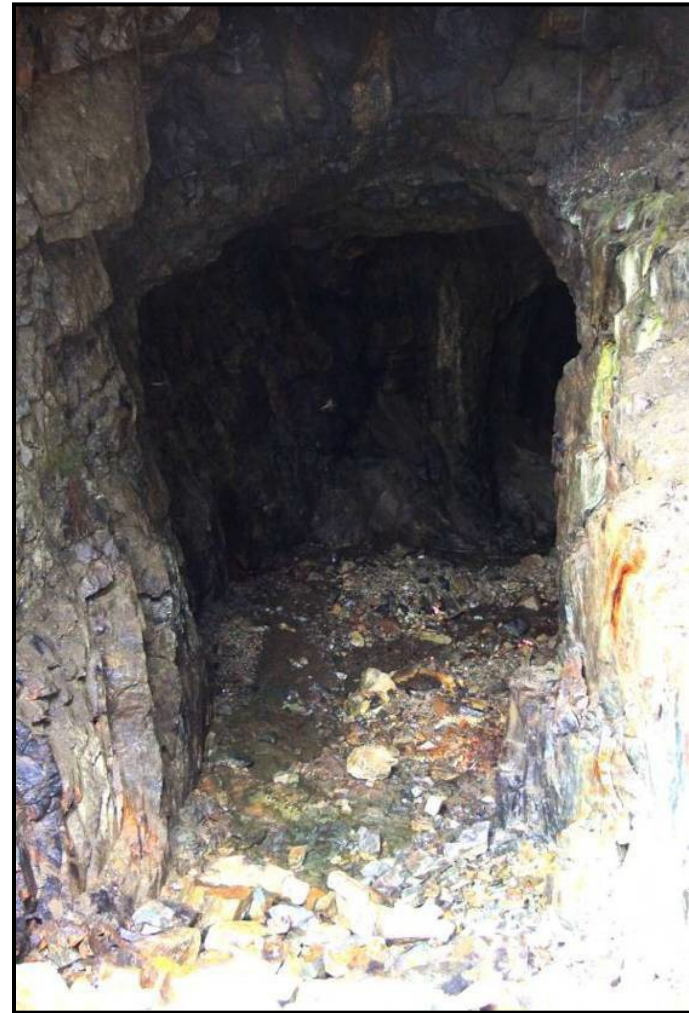
Photograph Looking South in at the 900-Foot Level Portal, showing water flowing from the rock pile which partially blocks the portal. (The photo also shows the adit bending toward the right (west) approximately 100 feet inside the portal.)
