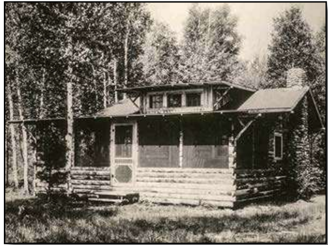
Figure 9—This 1934 photo of a recreation residence at the Deer Lake tract of the Chequamegon-Nicolet National Forest in the Eastern Region shows a shed-type dormer with windows that bring extra light to the interior of the building. The original photo caption: “Very good type of summer home construction.”
