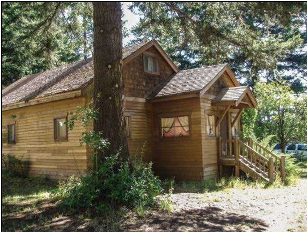
Figure 7—All of the siding on this 1917 recreation residence at the Chelminar Grotto tract of the Okanogan-Wenatchee National Forest in the Pacific Northwest Region was recently replaced with new siding in the same configuration as the original siding. Siding replacement is a major change, even when the new siding matches the original siding.
