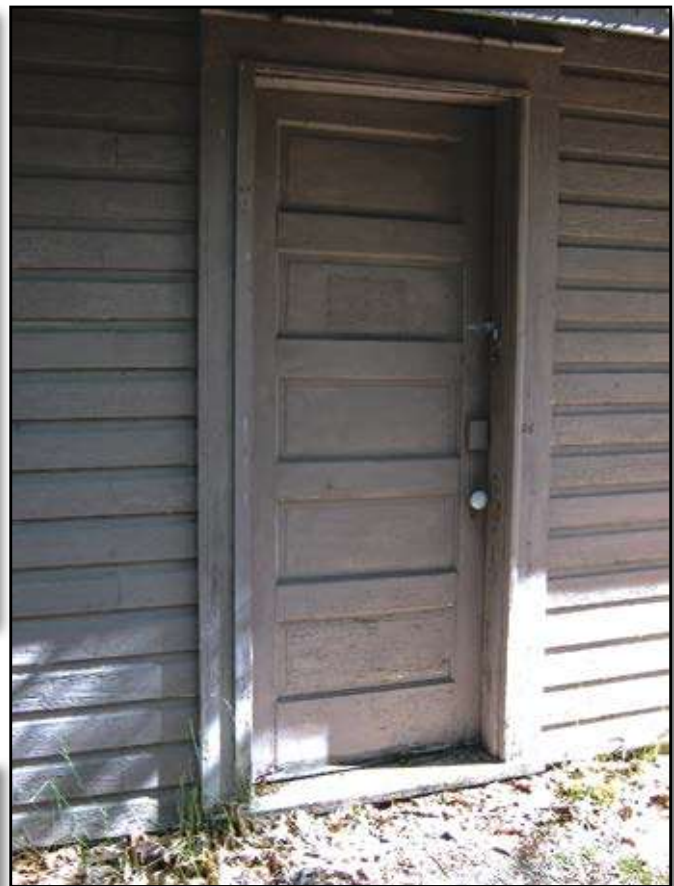
Figure 18—This rail and stile door is original to a mid-20th century recreation residence at the High Rollways tract of the Huron-Manistee National Forest in the Eastern Region.
