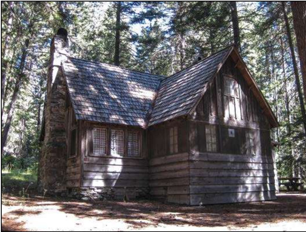
Figure 23—The foundation of this 1938 recreation residence at the Indian Creek tract of the Okanogan-Wenatchee National Forest in the Pacific Northwest Region raises the floor 1 to 3 feet above the gently sloping ground.
