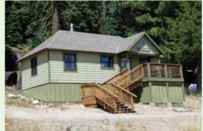
The Van Vleck bunkhouse is the last remnant of the Van Vleck Ranch site, which operated as a cattle ranch from the 1860's to the 1960's.
