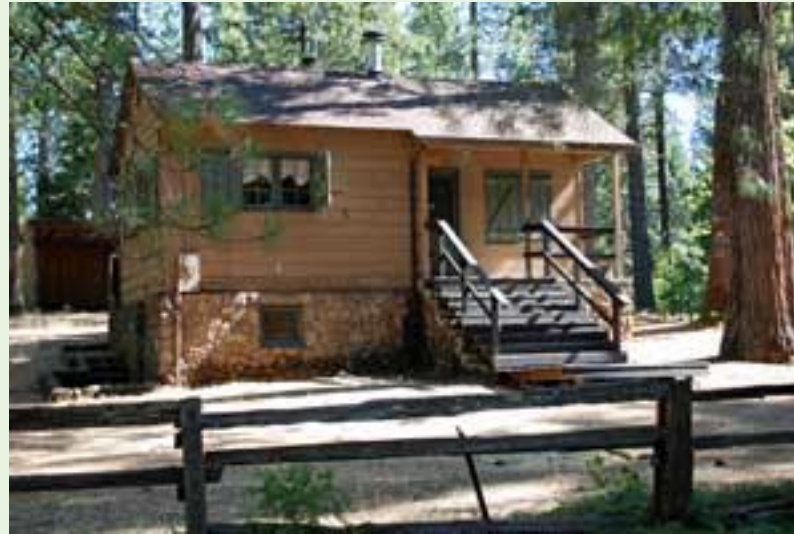
The Sly Guard Cabin, constructed in the early 1940's by the Forest Service, was a living quarters for rangers "on guard" in the Sly Park area.
