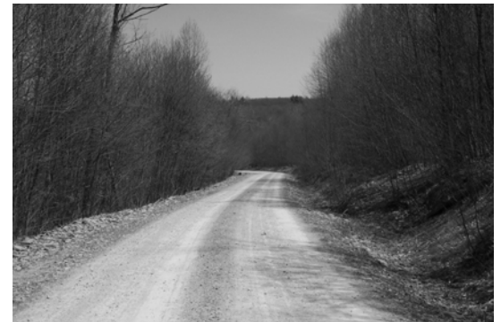
Figure 3-6. Maintenance Level 4 Road
