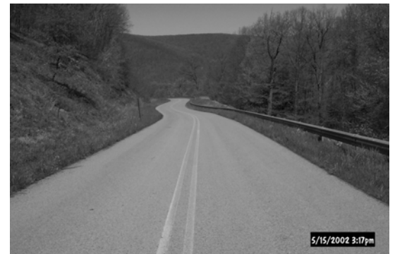
Figure 3-7. Maintenance Level 5 Road
