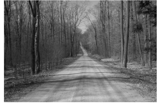
Figure 3-5. Maintenance Level 3 Road
