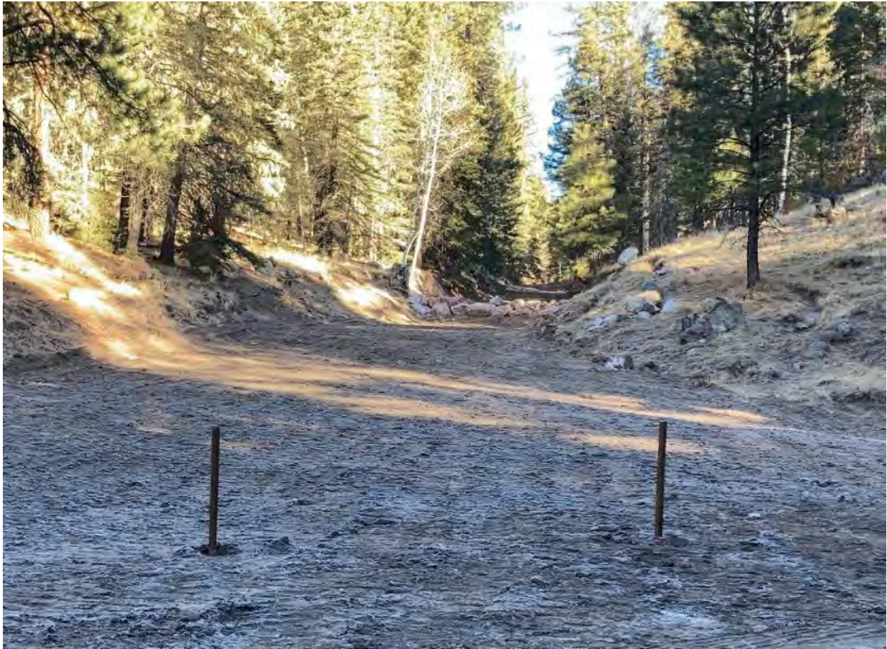
Fig. 1.10. Pipe rail (in progress) and erosion control structure in Mushroom Basin
