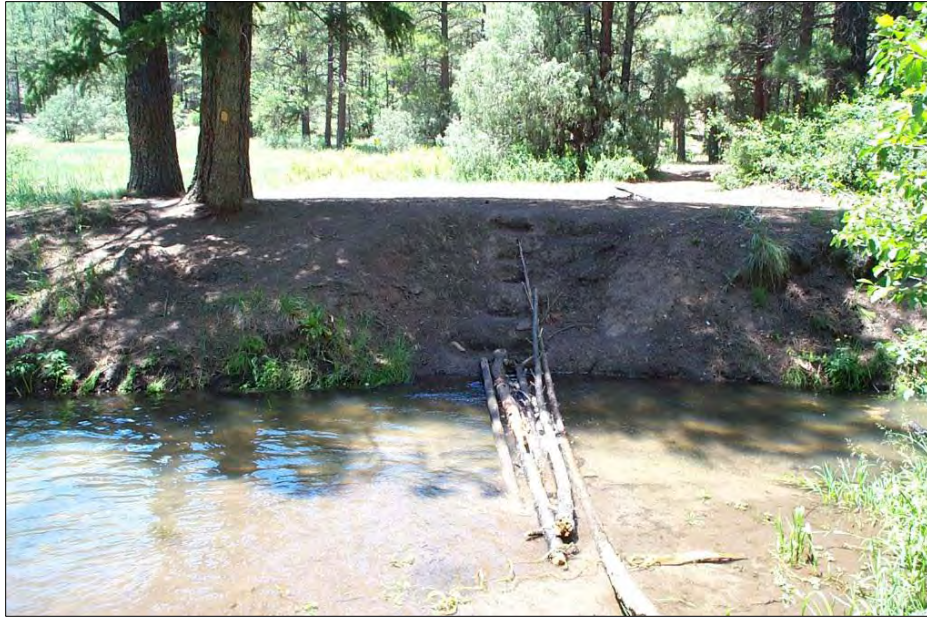
Figure 55. Dispersed campsite causing bank erosion on Rio Cebolla Reach 1, with wood being used to create a stream crossing
