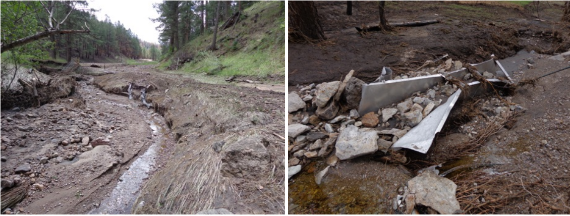
Figure 6— Pictures of left erosion from Thompson Ridge fire, right flume in lower Redondo destroyed by post fire erosion.
