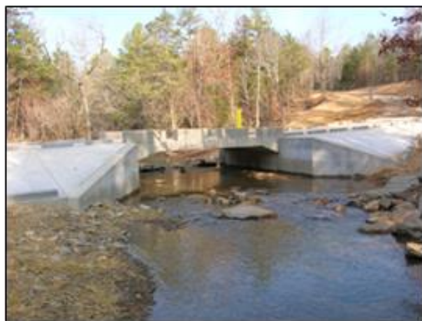
Replacement crossing on North Fork Cedar Creek for fish passage
