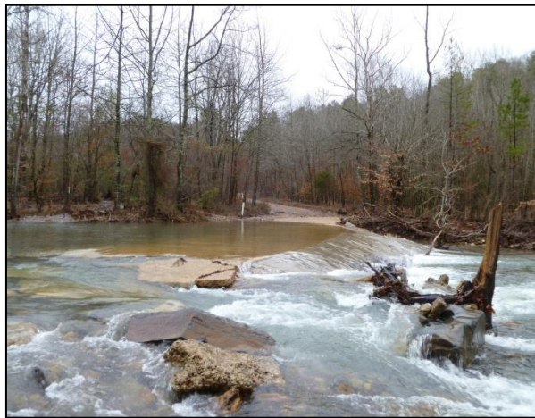
Original Brushy Creek FDR 140 Crossing AOP blockage under high water.
