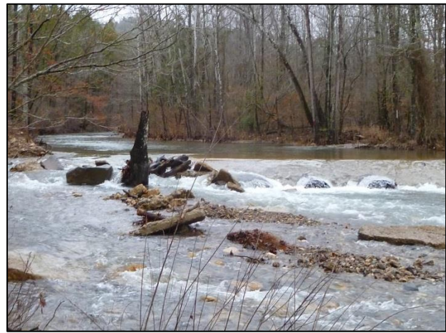
Original Brushy Creek FDR 140 Crossing AOP blockage under high water.
