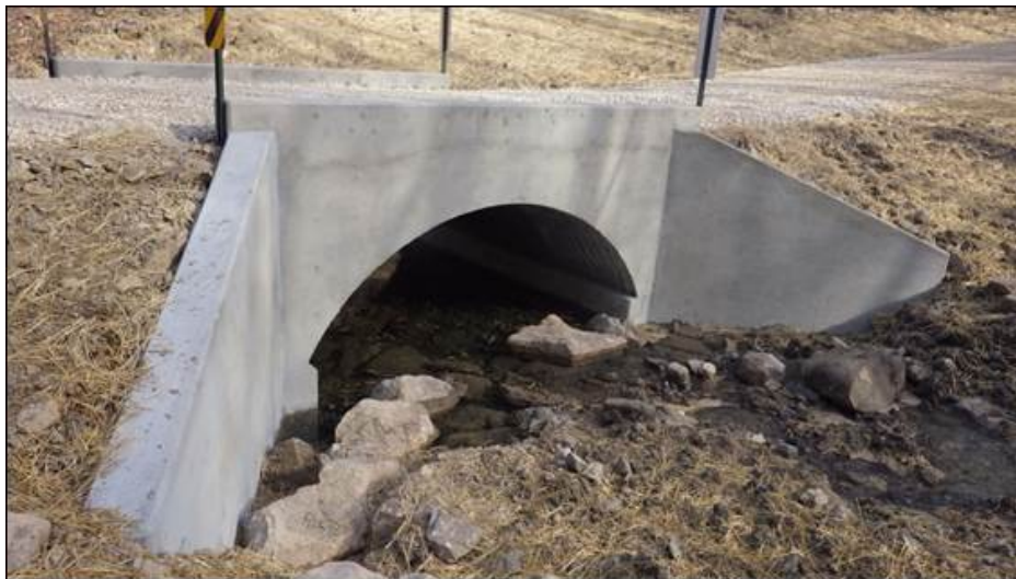
FDR 177 Replacement Crossing for Aquatic Organism Passage
