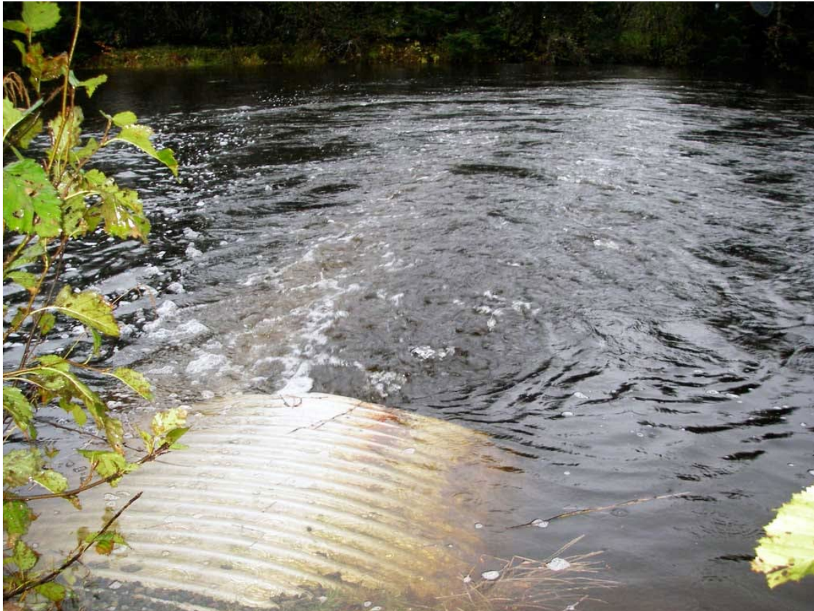
Figure 8. Flooded culvert planned for replacement on the Copper River Delta
