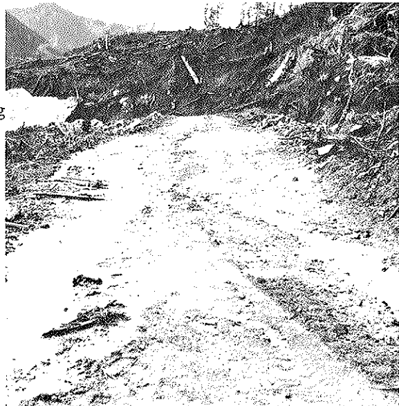
Figure 21 - Cutbank raveling on Soil 24.
