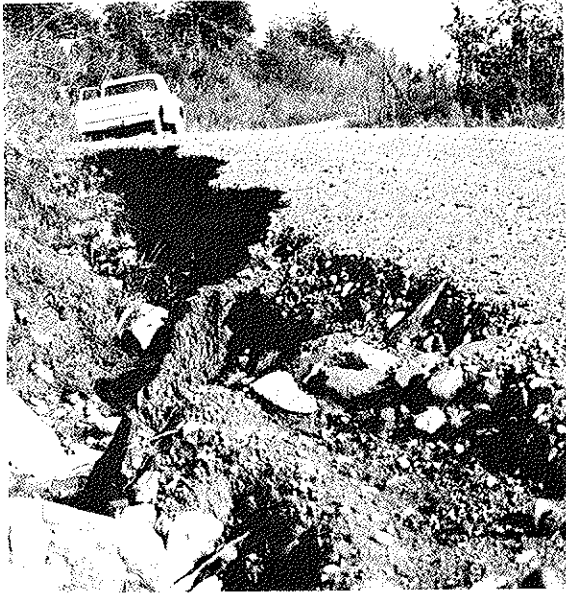
Figure 23 - Ditch erosion.
