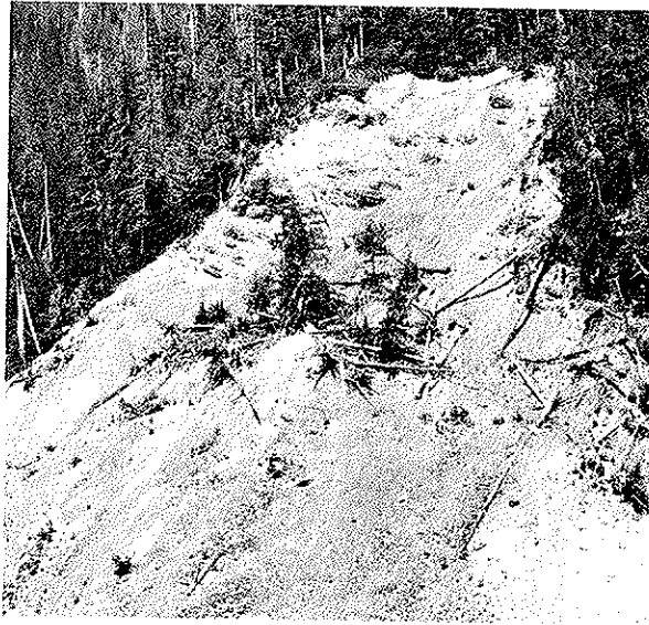
Figures 29 & 30 - Cutbank failures in unstable soils.
