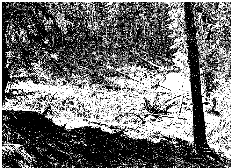
Figure 43 - Failure in Mapping Unit 35.
