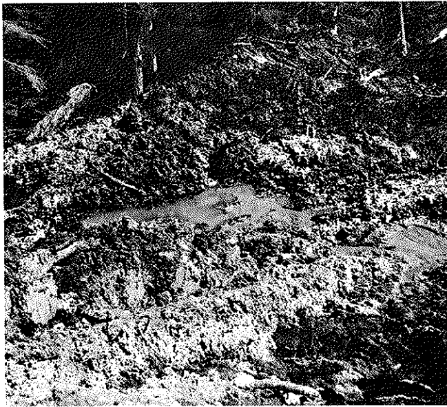
Figure 33 - Muddiness from wet weather road construction.
