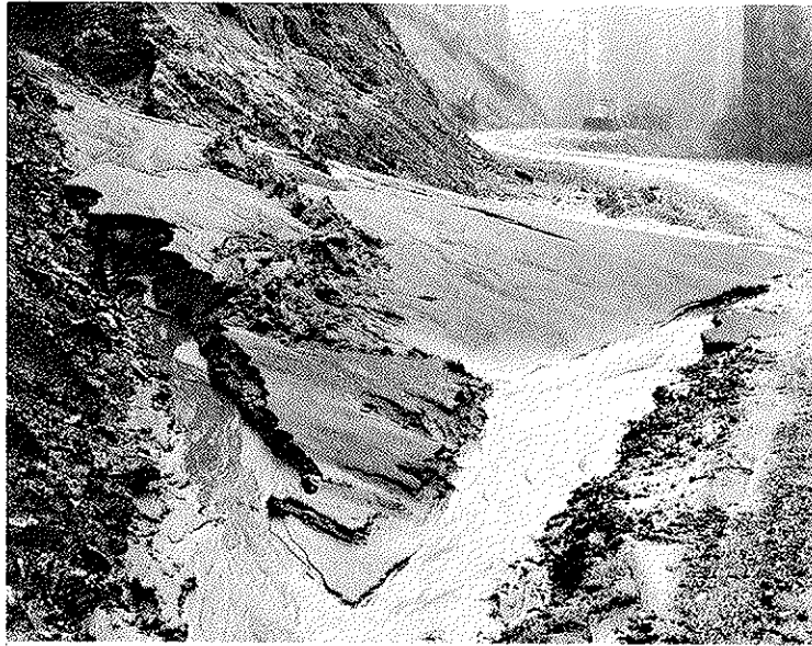
Figures 50 and 51 - Severe erosion in Soil 18.
