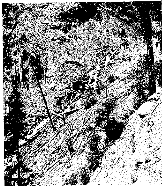
Figure 19 - Sidecast waste damage.
