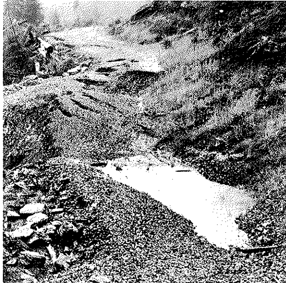
Figures 44 & 45 - Road prism failures in Mapping Units 34 and 35.
