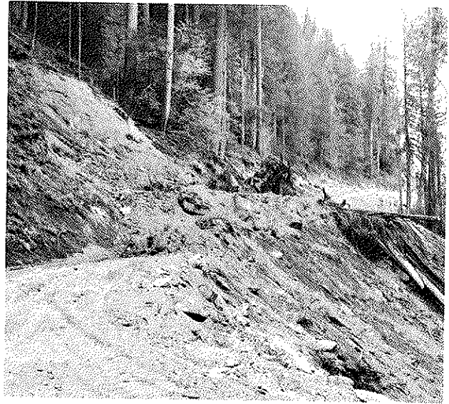
Figures 29 & 30 - Cutbank failures in unstable soils.
