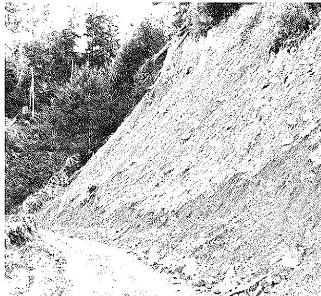
Figure 40 - Cutbank Raveling.
