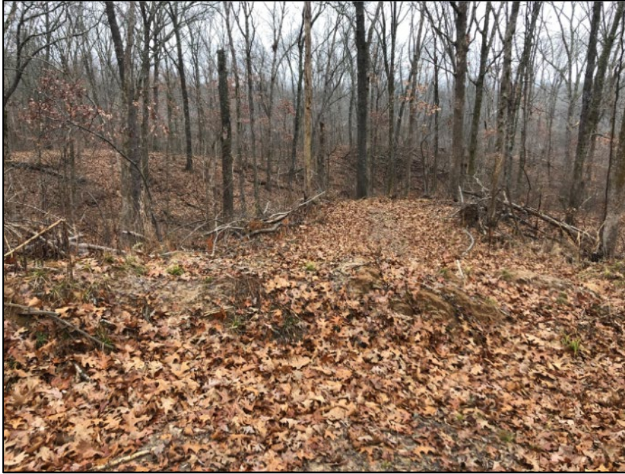
Figure 4 - Water bar installed at Kinkaid Salvage
