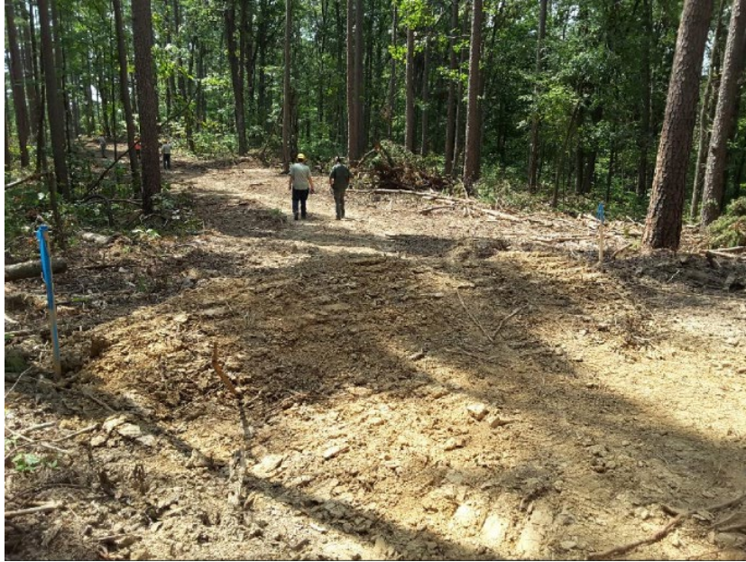
Figure 8-Photo of a water bar soon after Purchase Unit 1 was closed at Copperhead Road.
