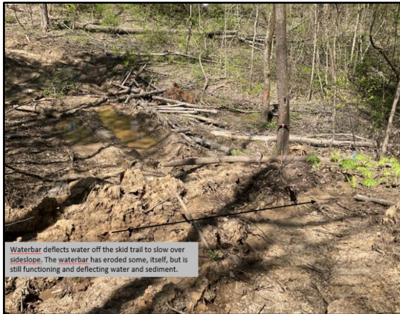
Figure 6-The photo shows a water bar deflecting water and sediment off the skid trail and down the slope to dissipate
