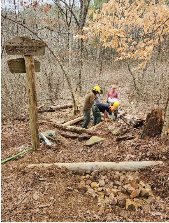
Figure 44-Trail tread and drainage feature maintenance
