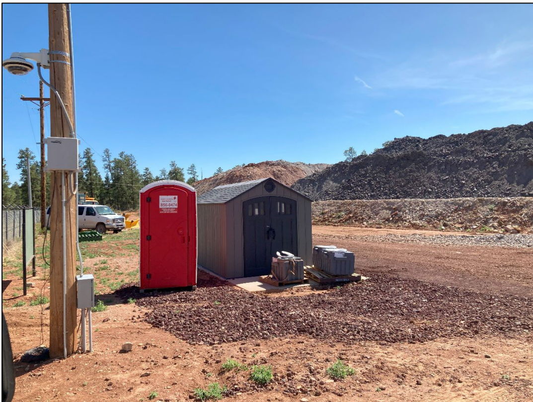
Photo 26 – Installed shed to be used by Navajo Nation. (May 23)
