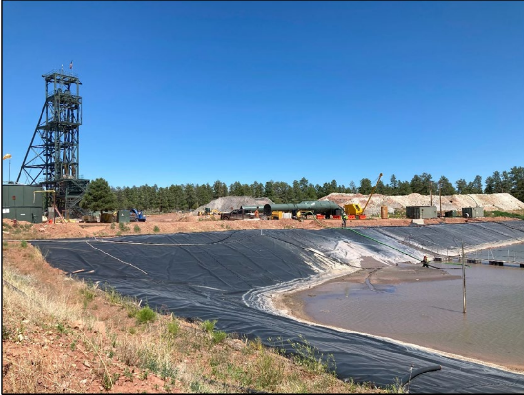
Photo 11 – Non-stormwater impoundment undergoing maintenance. (Jun. 23)
