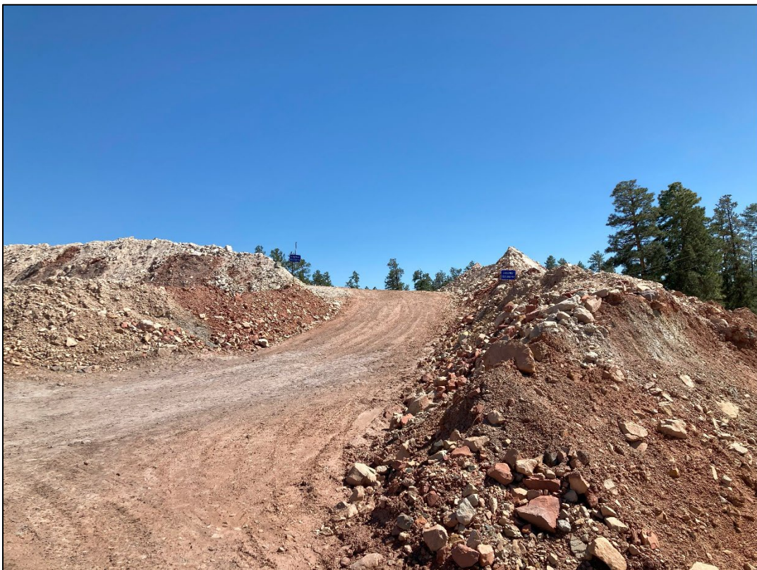
Photo 16 – Entrance of development rock stockpile. (May 23)
