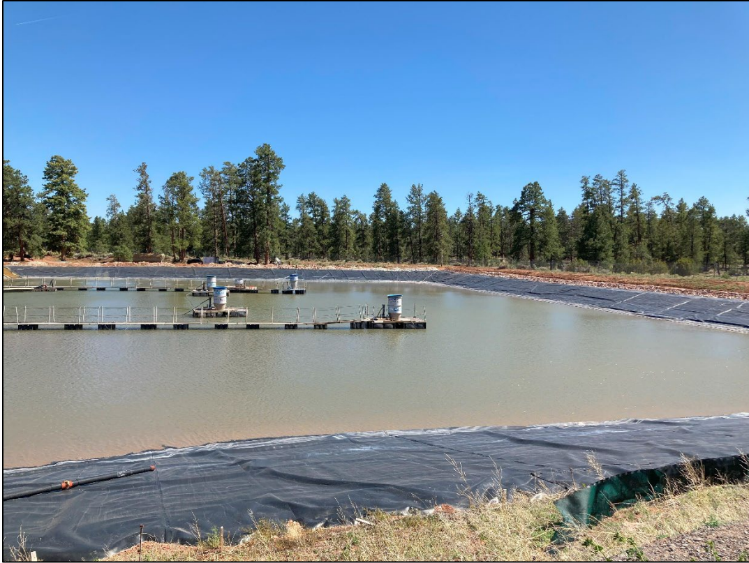
Photo 13 – Non-stormwater impoundment. All evaporators were offline. (May 23)
