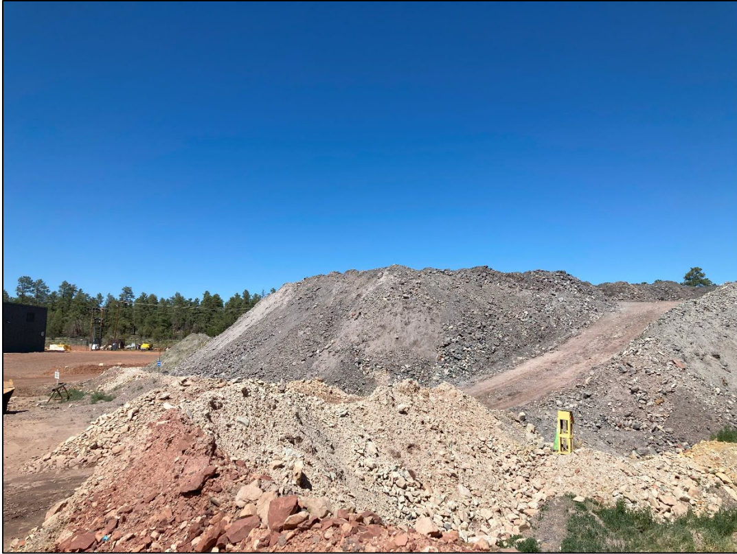
Photo 21 – Overlooking the ore pad from the entrance to the development rock stockpile, facing NE. (Jun. 23)
