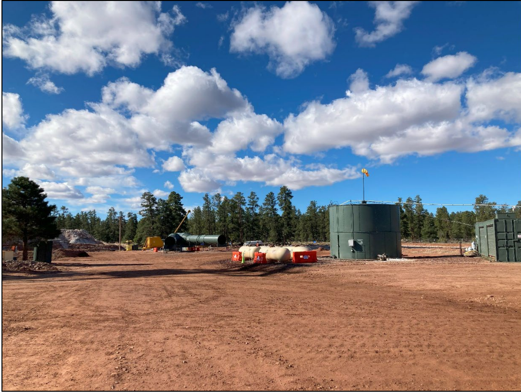
Photo 5 – Overlooking propane tanks, ventilation shaft and water storage tanks. (Apr. 29)
