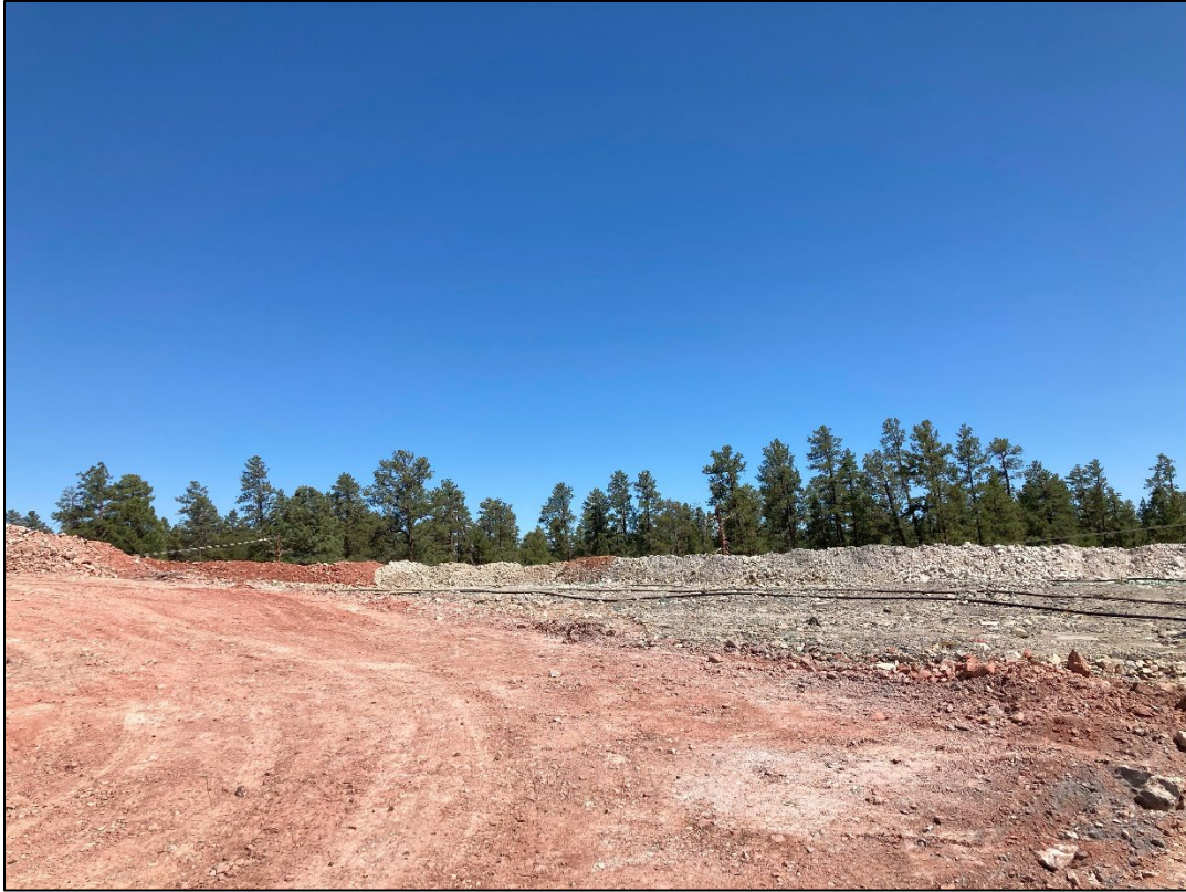
Photo 19 – Overlooking central area within development rock stockpile. (Jun. 23)
