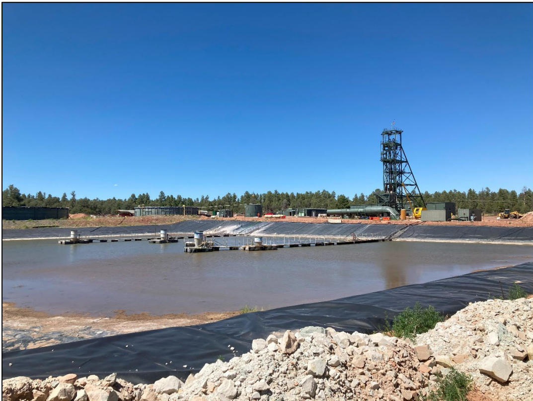
Photo 14 – Overlooking non-stormwater impoundment, facing NE. All evaporators were offline. (Jun. 23)
