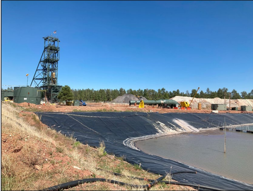
Photo 15 –Ventilation shaft undergoing maintenance. (May 23)
