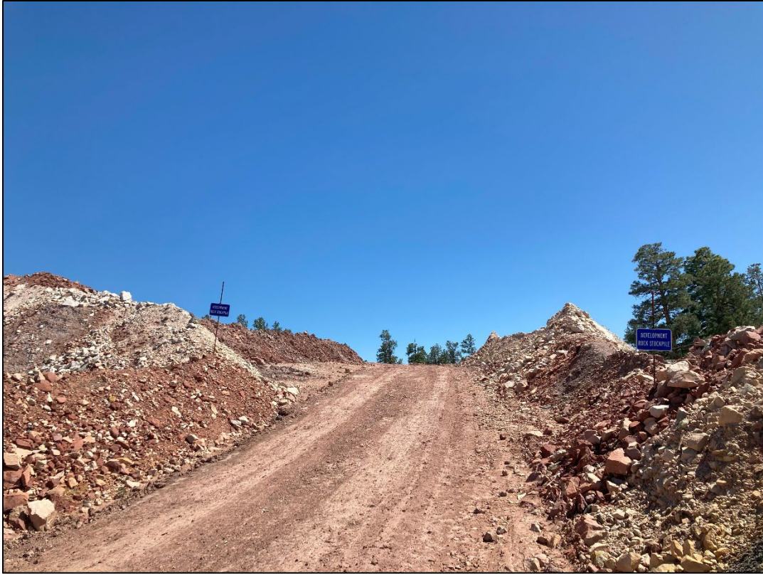
Photo 17 – Entrance of development rock stockpile. (Jun. 23)
