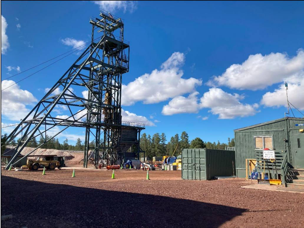
Photo 1 – View of the headframe from office trailer, facing south. (Apr. 29)
