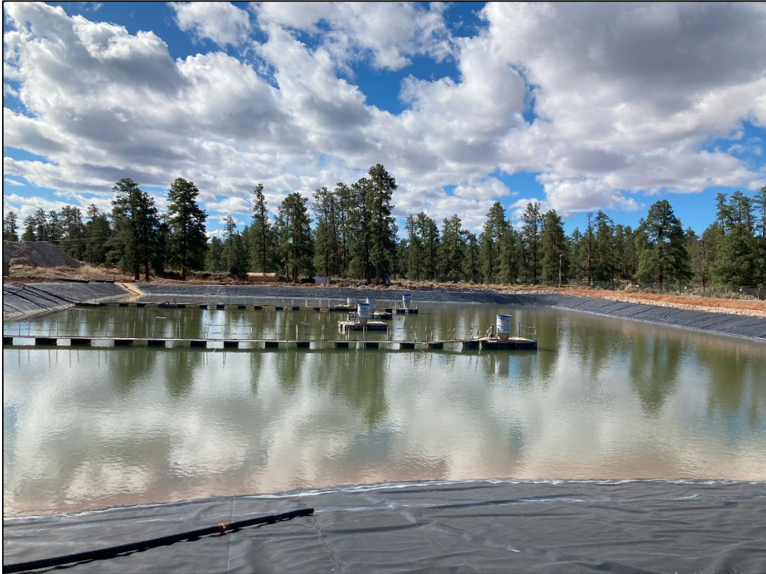
Photo 12 – Overlooking the non-stormwater impoundment. All evaporators were offline. (Apr. 29)
