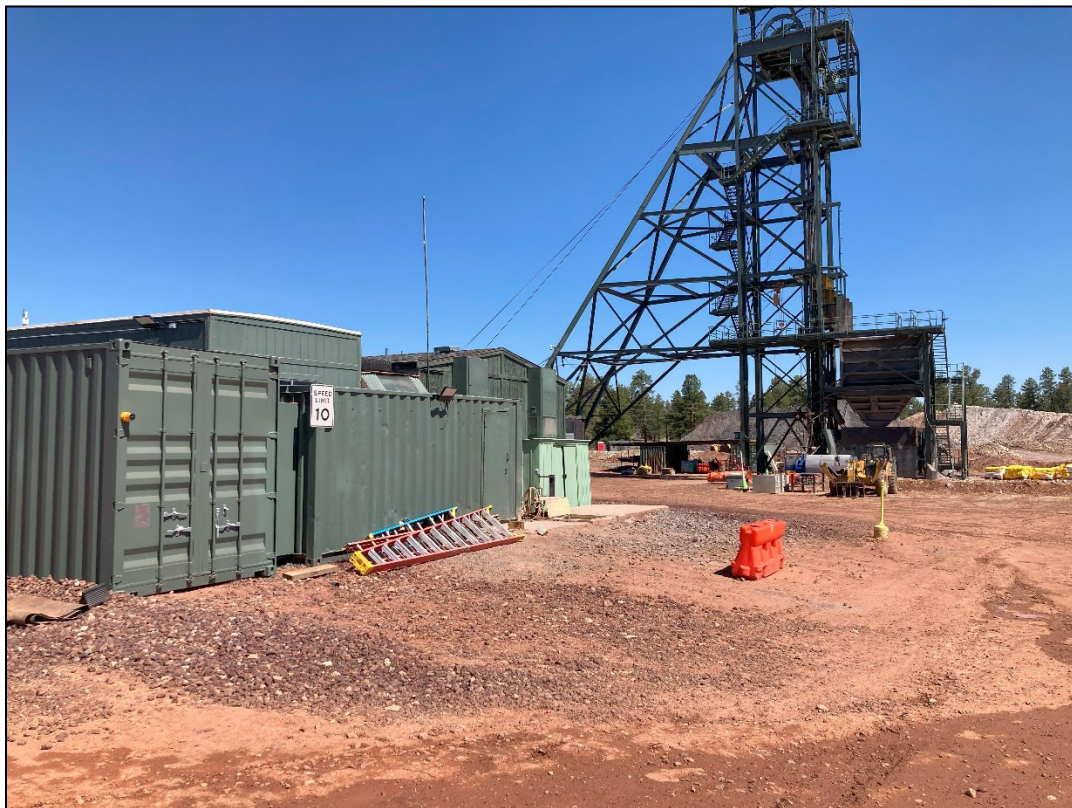
Photo 4 – Conex box storage for gear near the office building. (May 23)
