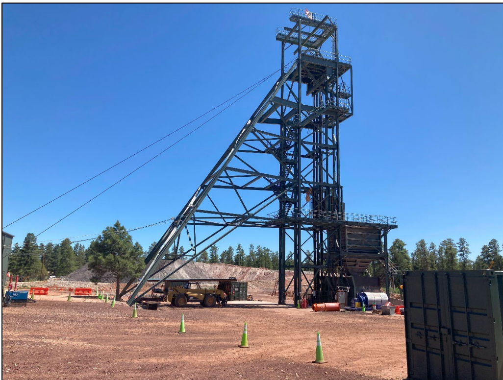
Photo 2 – Additional view of the headframe from office trailer, facing south. (Jun. 23)
