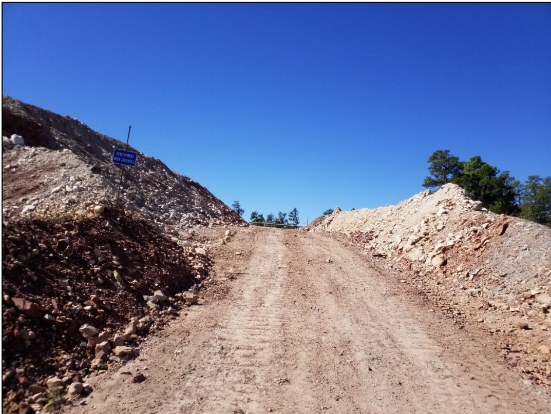
Photo 16 – Entrance of development rock stockpile. (July 30)
