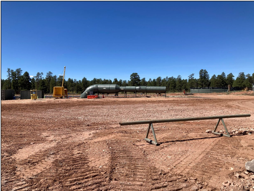
Photo 10 – After earthwork, overlooking the area where rainwater catchment previously existed. (Sept. 11)
