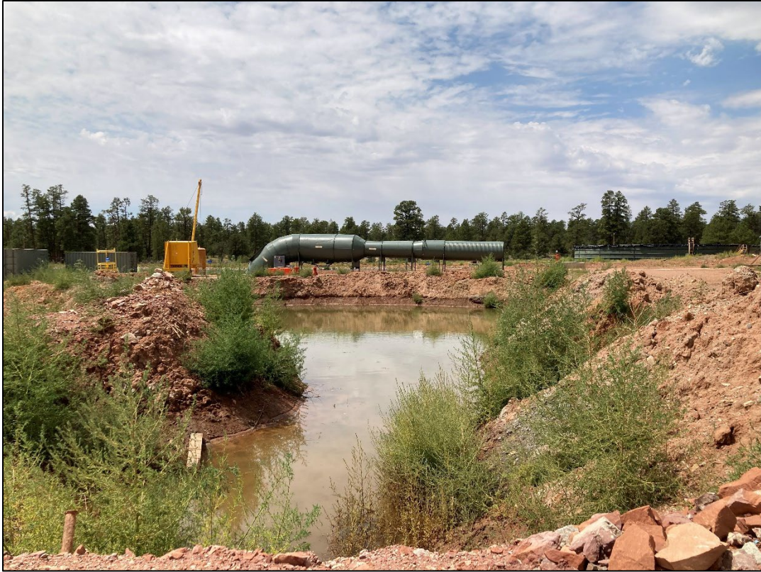
Photo 9 – Before earthwork, overlooking the central rainwater catchment, facing southwest. (Aug. 22)
