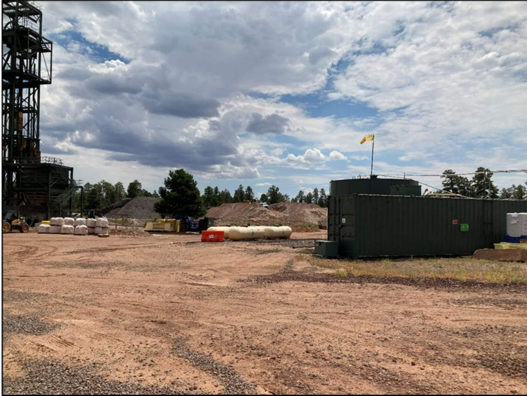
Photo 3 – Overlooking propane tanks near the center of the mine site. (Aug. 22)
