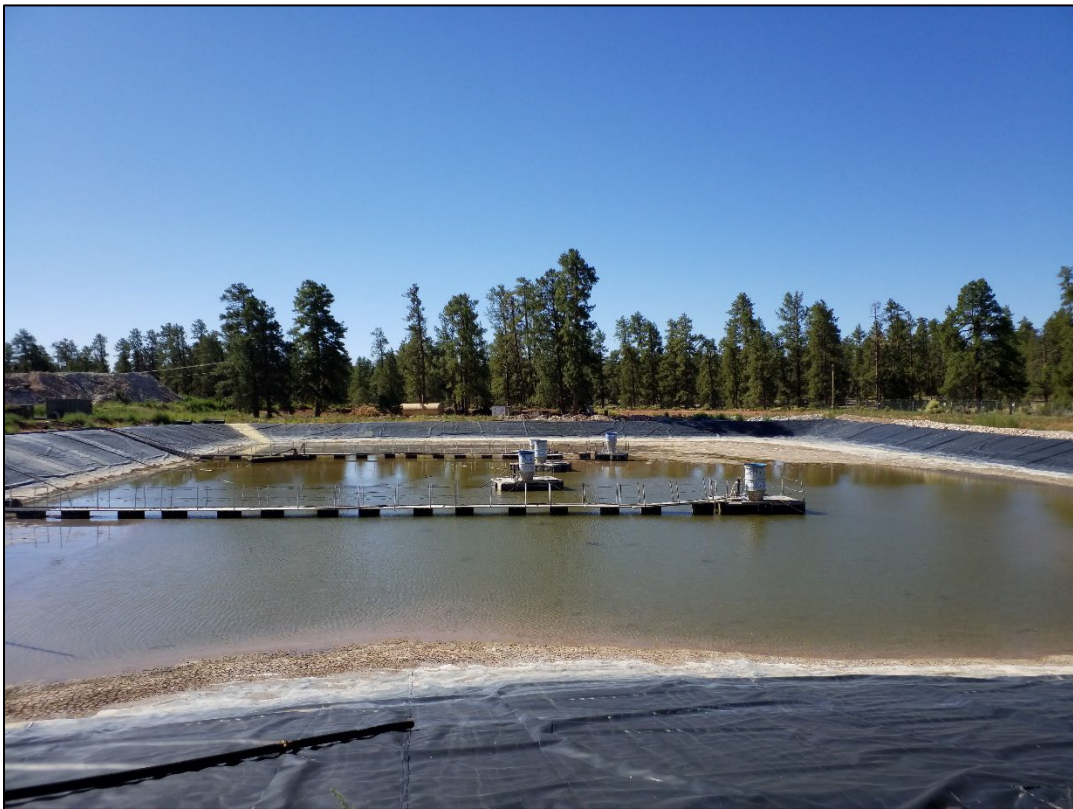
Photo 12 – Overlooking the non-stormwater impoundment. All evaporators were offline. (July 22)
