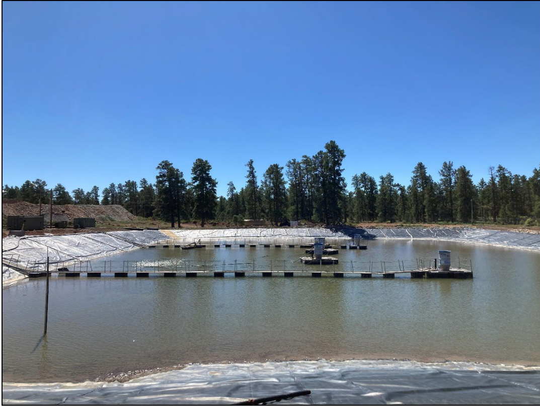
Photo 13 – Non-stormwater impoundment. All evaporators were offline. (Sept. 11)
