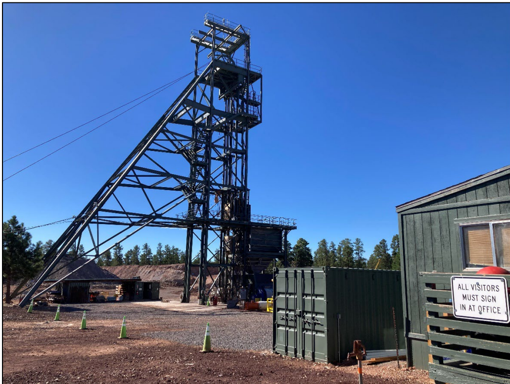
Photo 2 – Headframe from office trailer, facing south. (Aug. 22)
