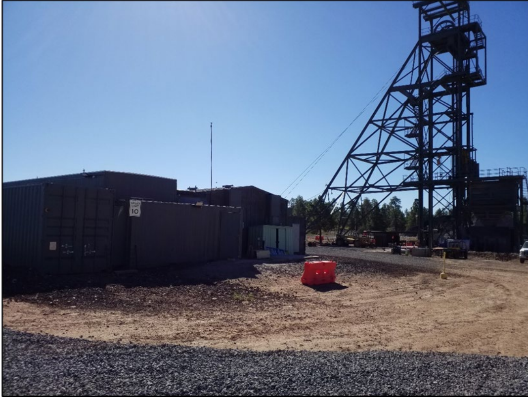
Photo 5 – Conex box storage for gear, adjacent to office buildings. (July 30)
