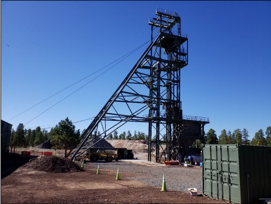
Photo 1 – View of the headframe from office trailer, facing south. (July 30)
