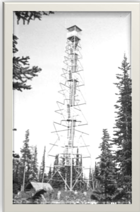
Elk Summit Lookout, 1952 This 100' steel Aermotor tower with a 7' x 7' cab was built in 1934. It is located six miles NW of Elk City on the Red River Ranger District.
