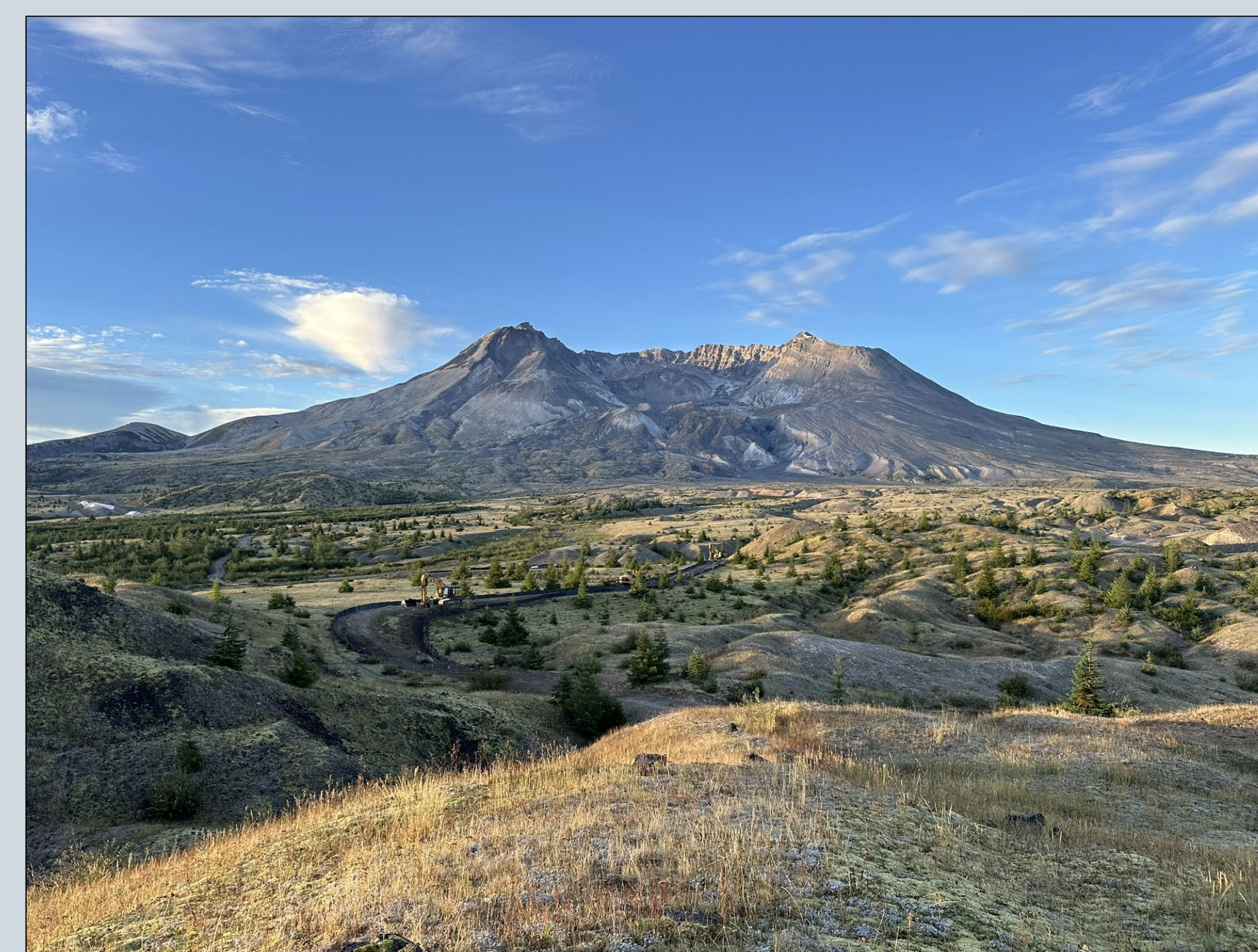
View of road, looking south to Mount St. Helens. Road, stockpiles, equipment visible.
