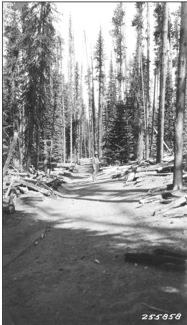
# 16 Chicken Hill Driveway – cleared to 10 ft. – Cost $100 per mile to widen to 30 ft.
