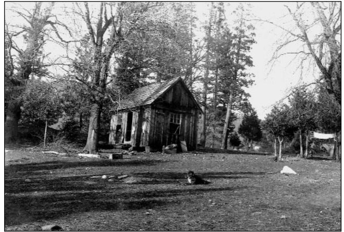
Figure 58—Former tool shed that served as the first forest entomology station office and laboratory for Miller at the supervisor's headquarters, North Fork, California, 1920s.
