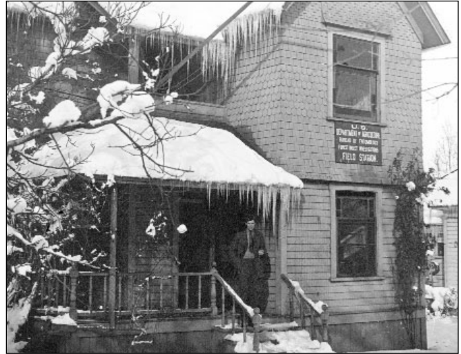
Figure 52—From 1919 to 1924, the station was housed in the residence building (shown at right) in the town of Ashland. This picture was taken in February 1920 following a heavy snow and cold snap in the Rogue River Valley. John Patterson is on the porch.
