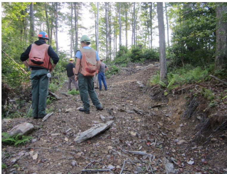
Figure 9. A steep skid trail lacking adequate mulching or surface protection
