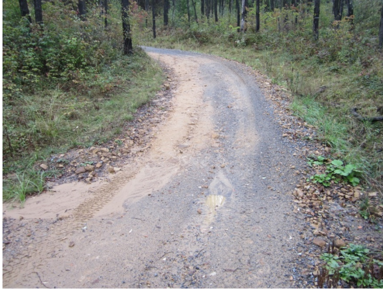
Figure 7. Sediment path flowing toward Red Lick Run resulting from a lack of defined leadoff ditches and inadequate trail maintenance
