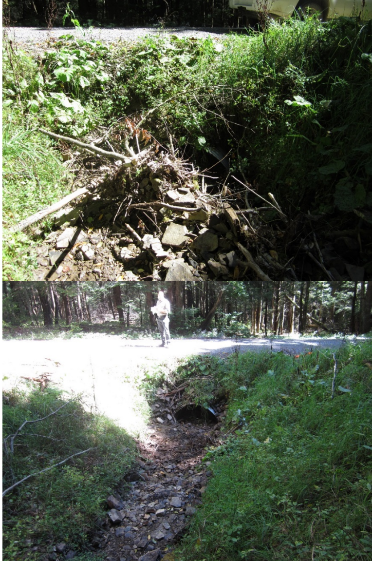
Figure 8. FR 119 culvert prior to culvert cleaning (top) and after cleaning of the inlet (bottom)
