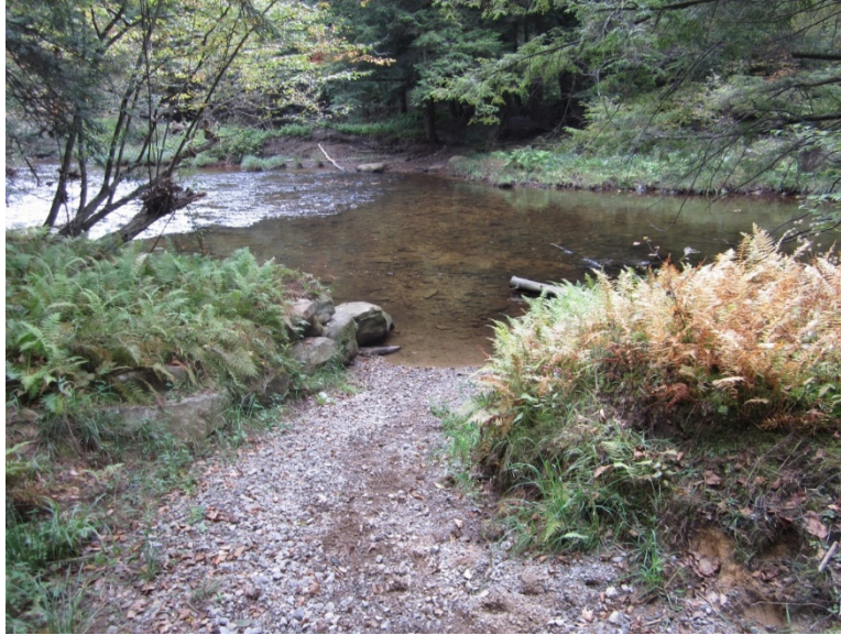
Figure 6. Armoring of ford approach at the Spring Creek Horse Trail
